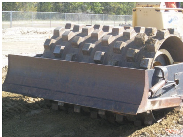
FIGURE 80 Compaction of a low plasticity clayey silt (CL-ML) using a sheepsfoot roller.
