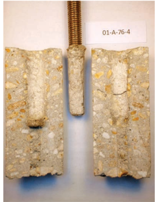
Figure 49. Typical adhesive bond failure.
