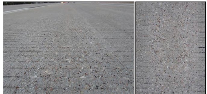
a) High-Pressure Water Blasting
