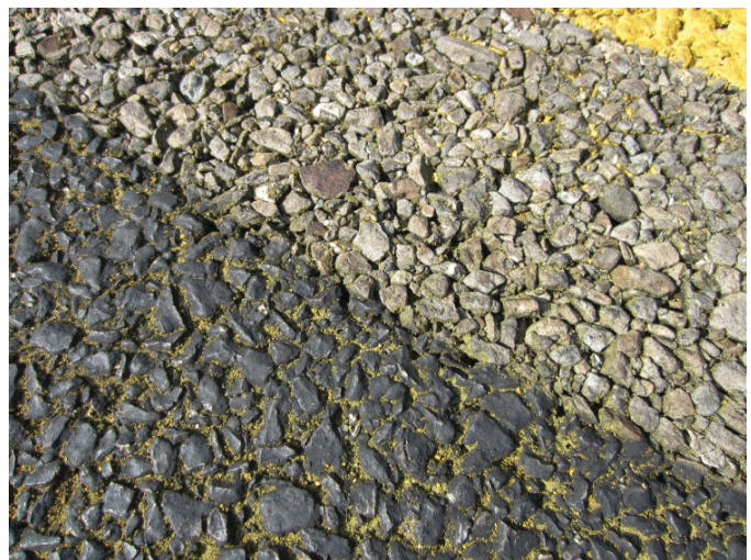
Figure 34. Water blasted thermoplastic on new asphalt surface (close-up).
