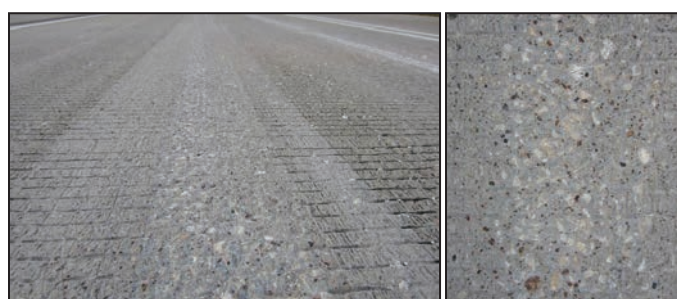
d) Combined Removal Flailing and High-Pressure Water Blasting
