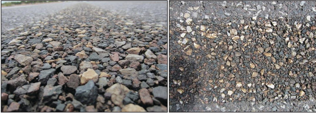
a) High-Pressure Water Blasting
