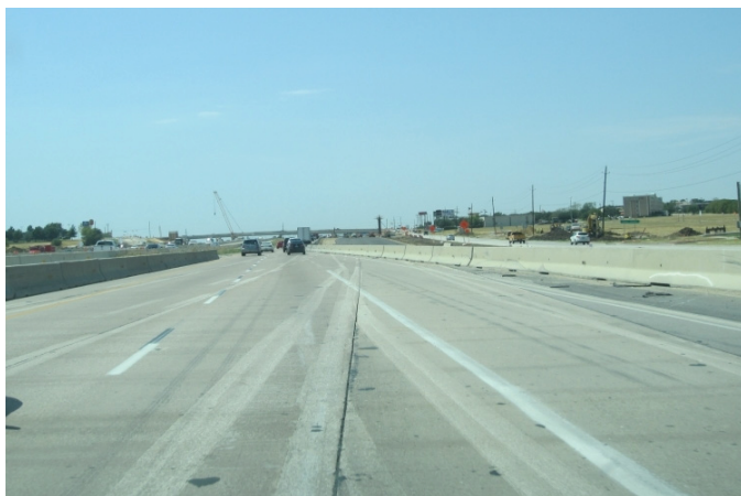
Figure 40. Ghost markings due to surface color changes near merge area.
