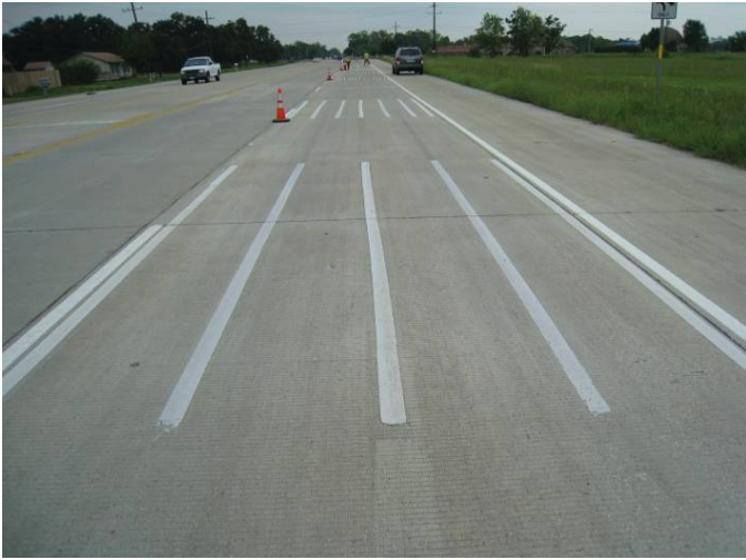
Figure 10. Pavement marking test deck on PCC surface.
