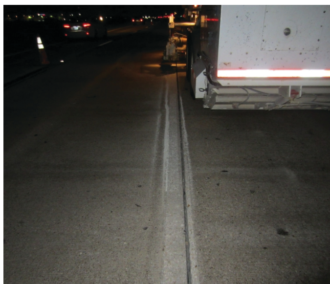
Figure 30. Full-size flailing truck removing thermoplastic on PCC (behind).
