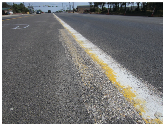
Figure 37. Hand flailed thermoplastic on asphalt surface.
