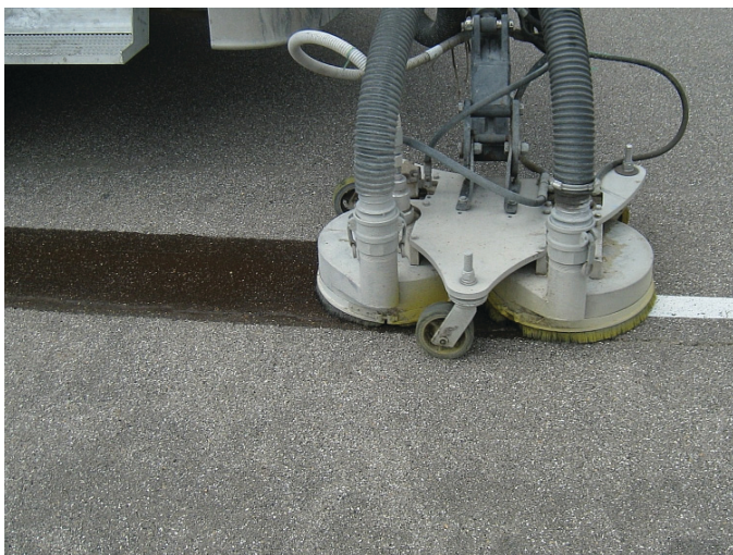
Figure 38. Water blasting paint on surface treatment.
