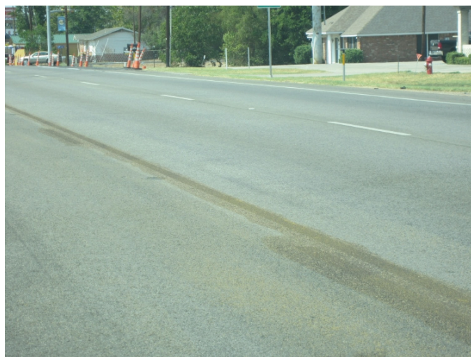
Figure 35. Water blasted thermoplastic on asphalt surface (wide view).
