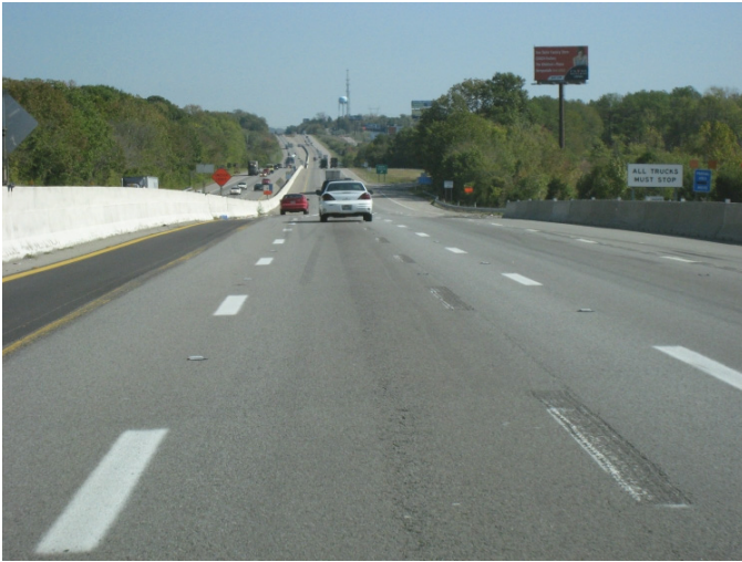
Figure 44. Removed lane lines and wider markings.
