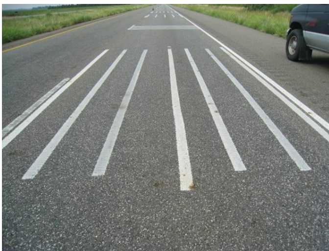
Figure 11. Pavement markings test deck on asphalt surface.
