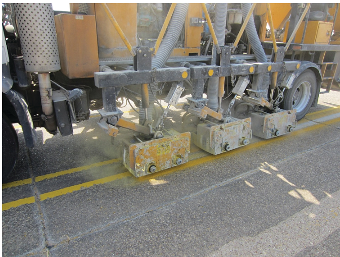
Figure 15. Flailing on PCC closed-course test deck.
