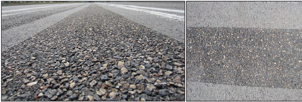
a) High-Pressure Water Blasting
