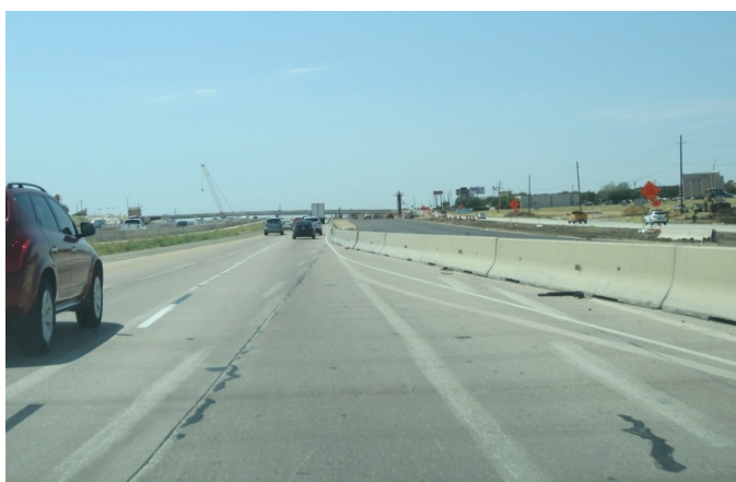
Figure 41. Ghost markings due to surface color changes at merge area.
