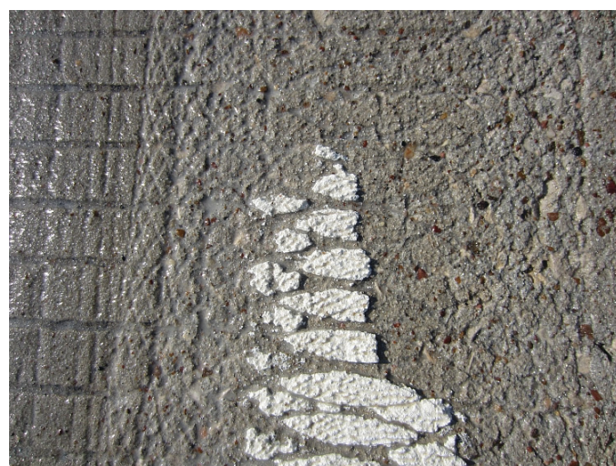
Figure 18. Close-up of high-pressure water blasting removal of MMA on PCC.
