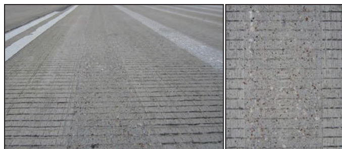
a) High-Pressure Water Blasting
