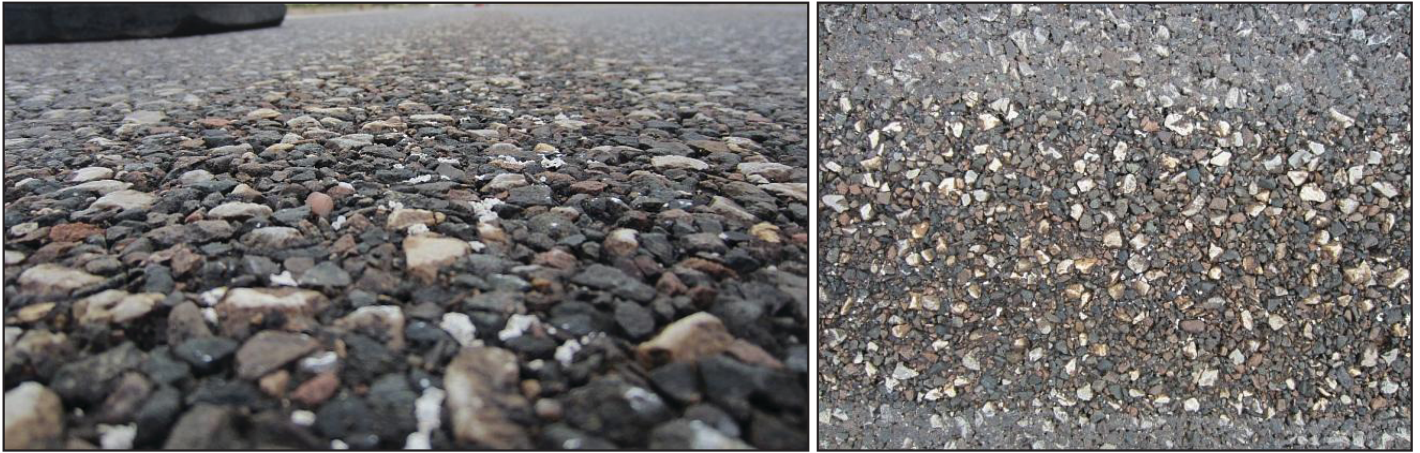
a) High-Pressure Water Blasting
