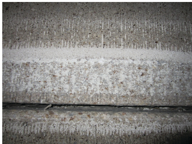
Figure 31. Flailing truck removal of thermoplastic on PCC (above).
