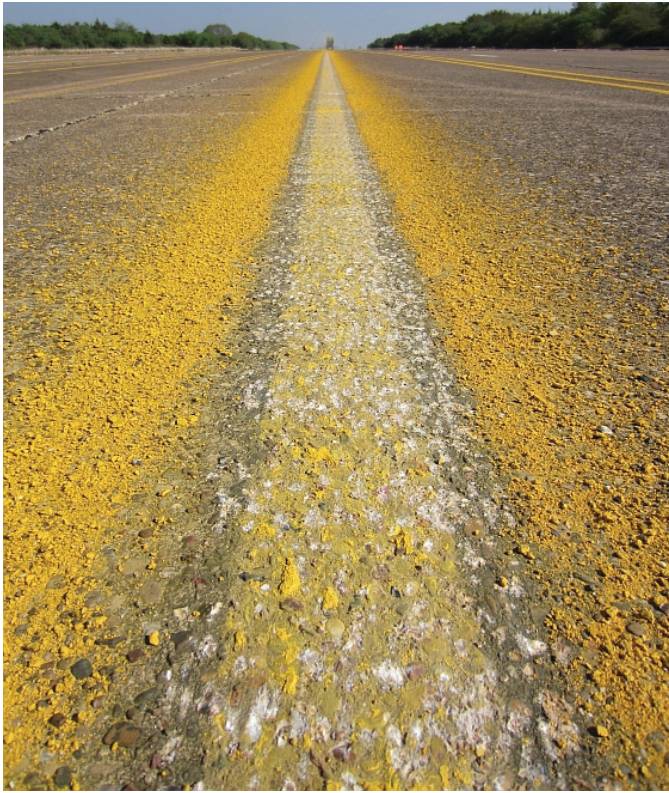
Figure 29. Combined removal remnants prior to high-pressure water blasting of thermoplastic on concrete.
