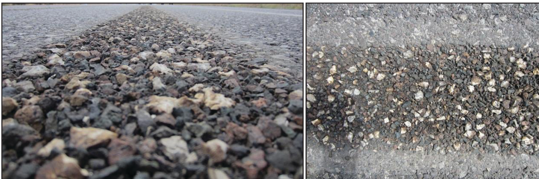
d) Combined Removal—Flailing and High-Pressure Water Blasting
