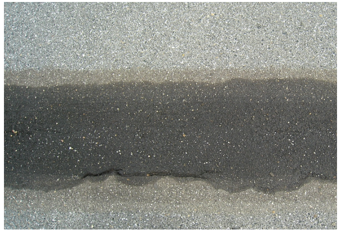
Figure 39. Removed area immediately after water blasting.
