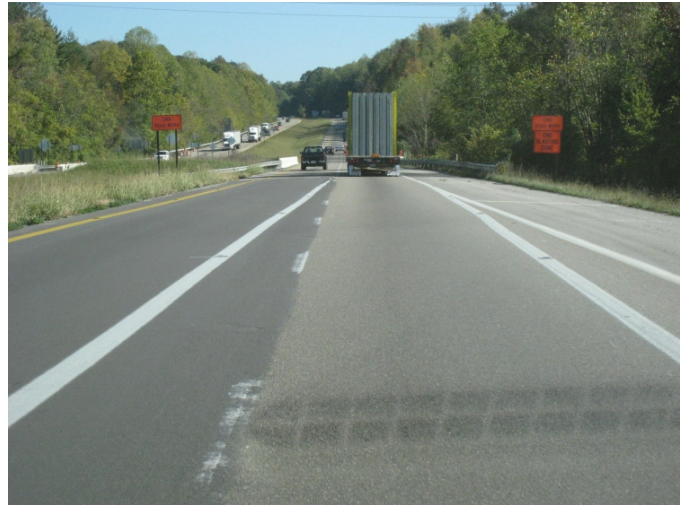
Figure 45. Wider and continuous markings in lane shifts.
