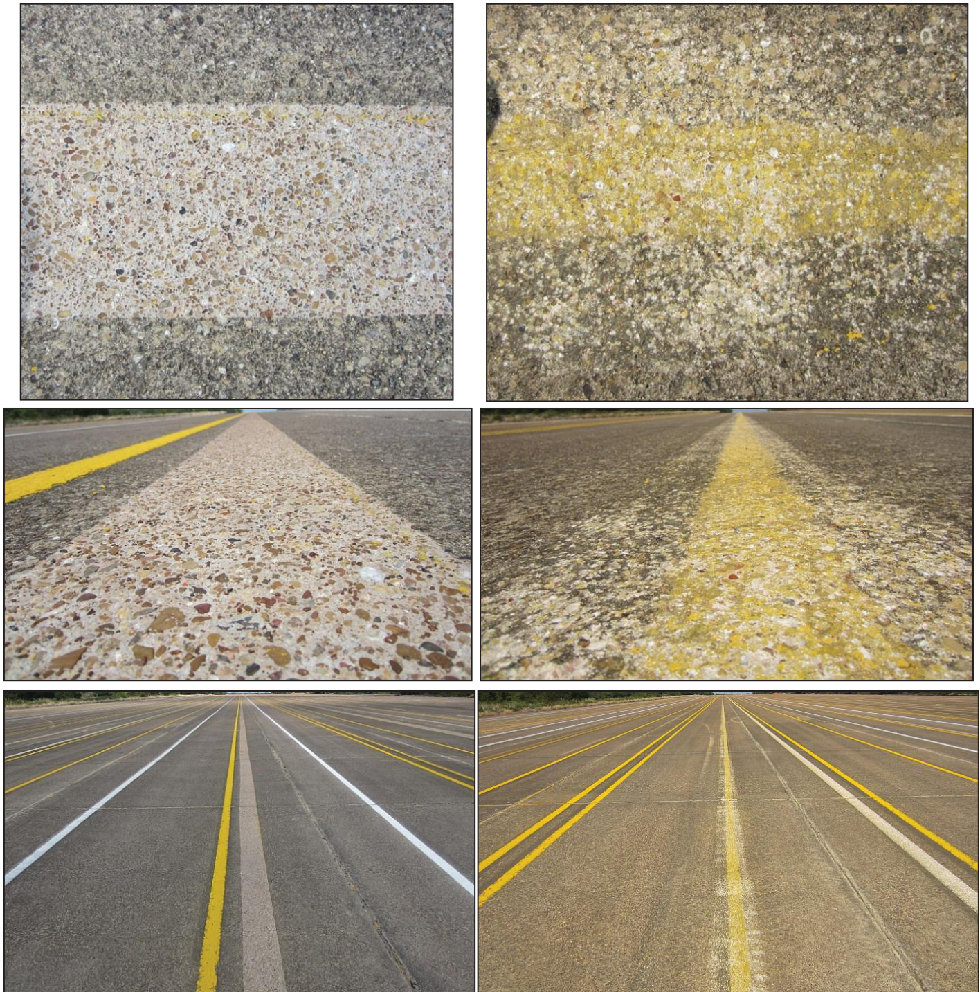
a) High-Pressure Water Blasting
