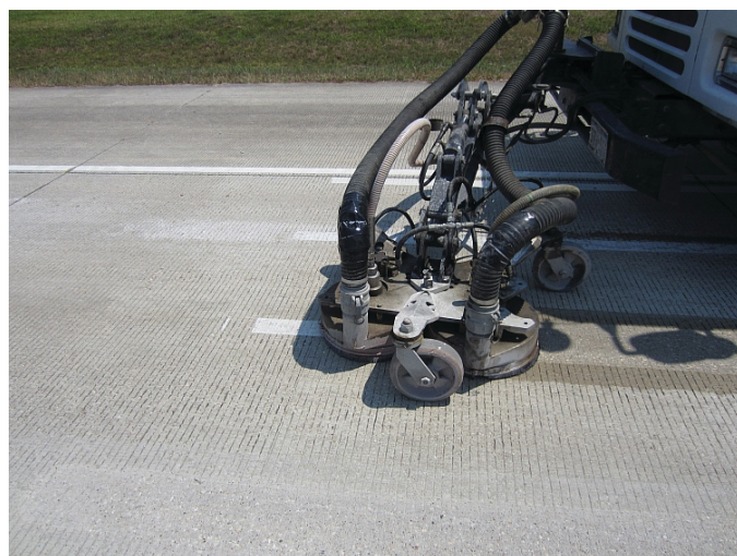
Figure 13. High-pressure water blasting on PCC test deck.
