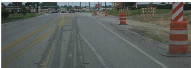
a) Ghost markings resulting from scarring and/or surface characteristic changes and incomplete marking removal.
