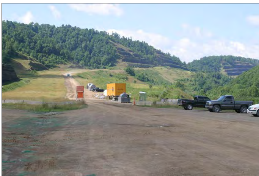
Figure 1.1. Construction access to ongoing activities on the Coalfields Expressway.
