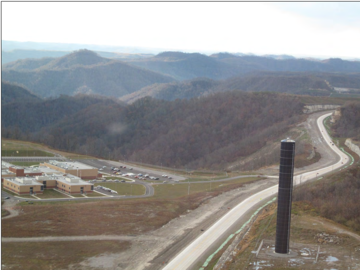
Figure 1.3. This section of the King Coal highway, planned to incorporate the Mingo Central Comprehensive High School, was opened with the new school and ready for 2011-2012 year.
