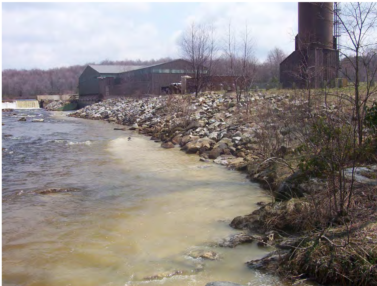
Figure 4.2. Limestone doser on the Blackwater River in Tucker County, West Virginia. Note the small impact area, and treatment resulting in some of the most well-known catch-and-release trout fishing opportunities in the state.
