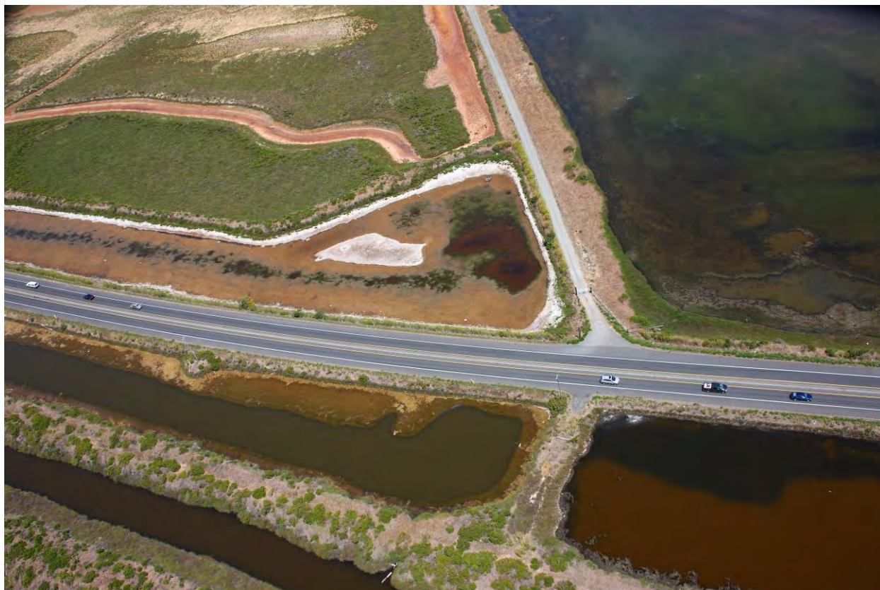
Figure 8.1. State Highway 37 traversing wetlands and fresh/brackish impoundments.
