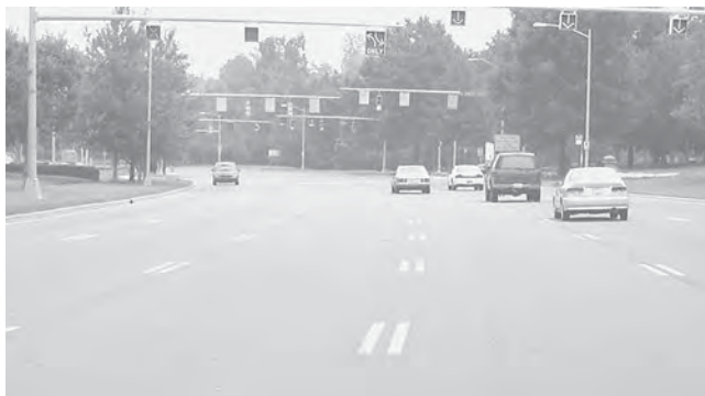
FIGURE 8 Example of reversible arterial lane in Charlotte, North Carolina. Source: NCHRP Synthesis 340 (Wolshon and Lambert 2004).
