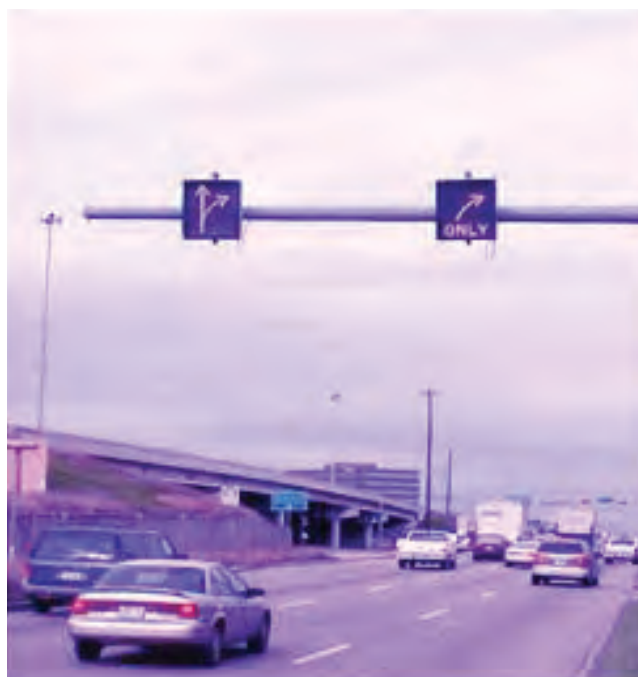
FIGURE 3 Example of dynamic turn lanes installation. Source: FHWA-HRT-06-095 (Urbanik et al. Coordinated Freeway and Arterial Operations Handbook , 2006).
