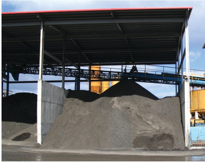
Figure 12. Covered stockpile to minimize moisture in RAP.
