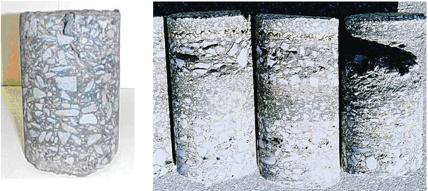
Figure 2. Roadway cores showing distressed layers: top-down cracking on left, stripping damage on the right.
