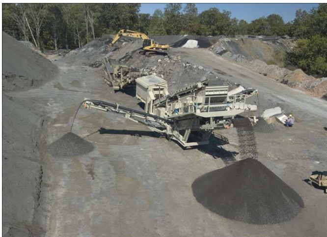
Figure 7. Excavator feeding material into a RAP crushing and screening process.
