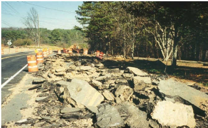
Figure 5. Pavement rubble from full-depth demolition of a roadway.
