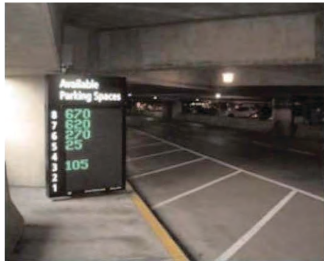
FIGURE 16 Sign in the parking structure directing traffic to open parking spaces (25). (Source: ACRP Report 52).
