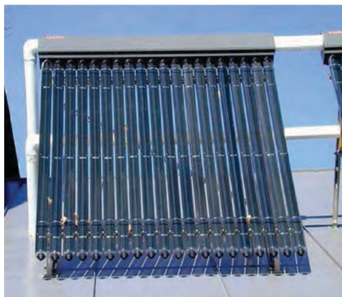
Figure 10-2. Evacuated-tube collector.
