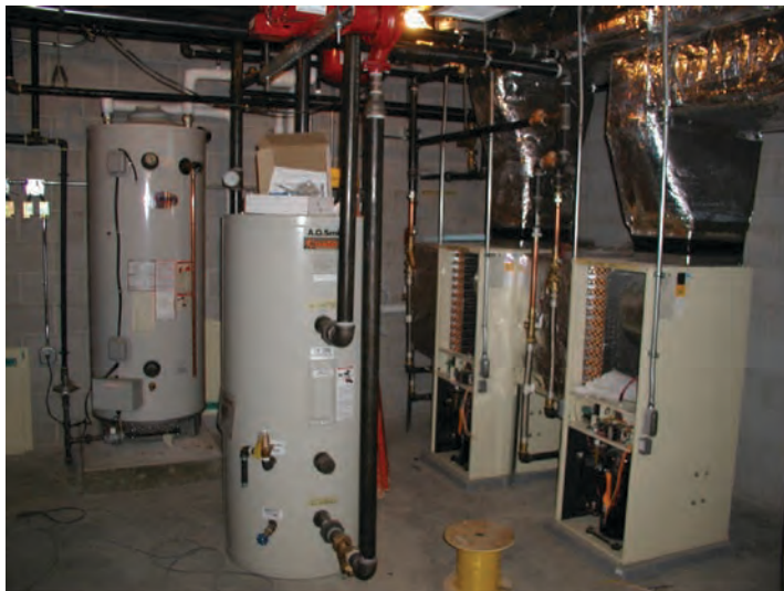
Figure 22-57. Two water-to-air heat pumps supply the office spaces.
