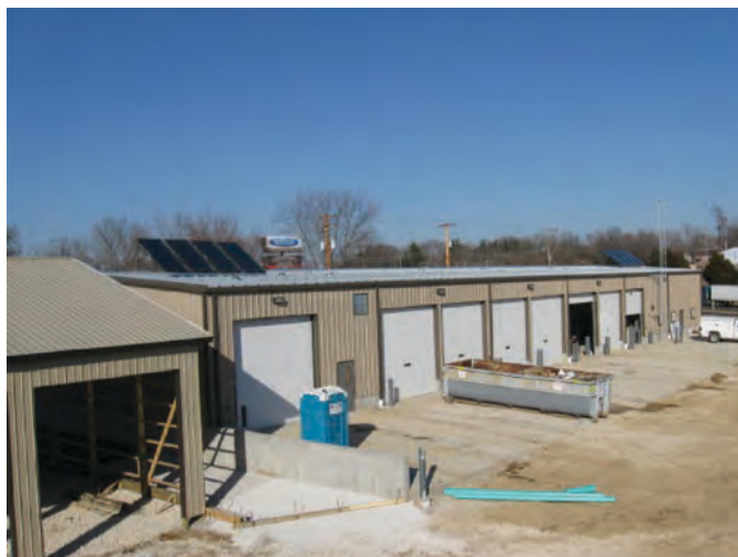
Figure 22-4. Solar collectors for water heating on each end of Building A.
