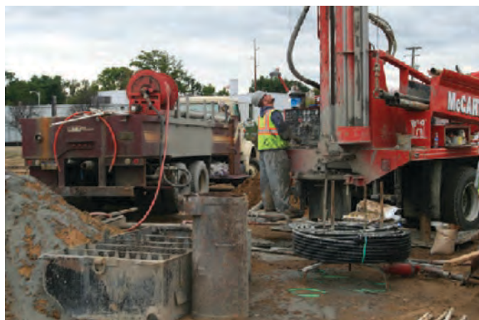
Figure 22-36. Construction of ground-source (geothermal) heat pump wells.
