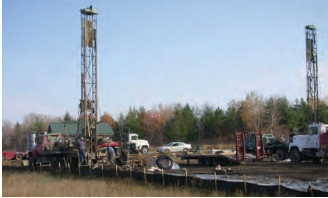
Figure 22-56. Drilling rigs during installation of vertical well field.
