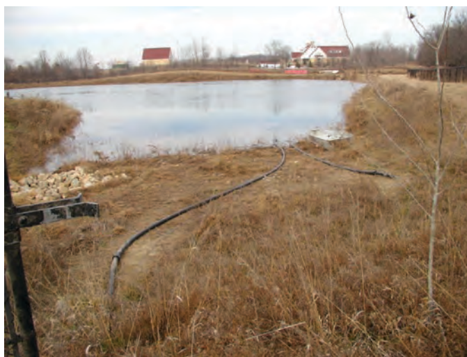
Figure 22-55. Pond with heat exchange piping.
