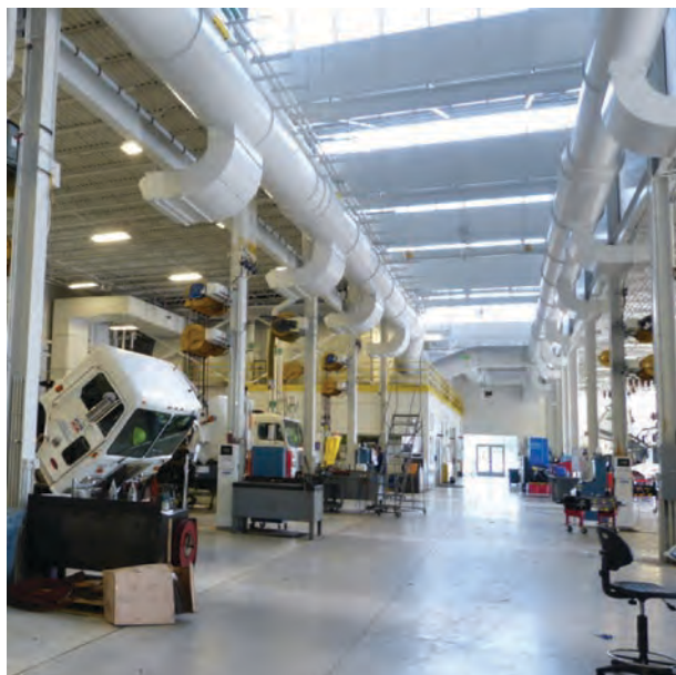
Figure 22-28. Daylighting looking toward light monitors.
