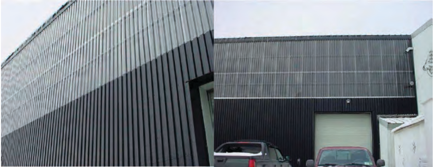
Figure 22-18. Completed two-stage SolarWall installation.
