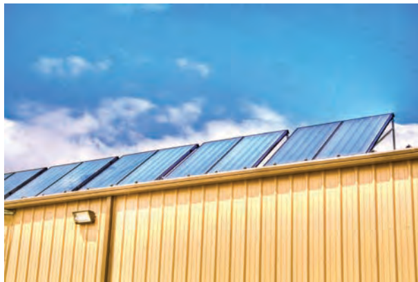
Figure 22-7. Solar air collector array.
