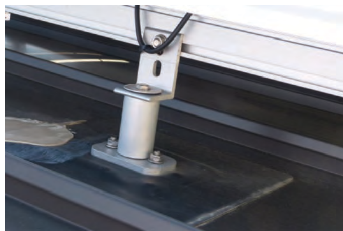
Figure 22-31. Penetrating mounting—standing seam metal roof installation.
