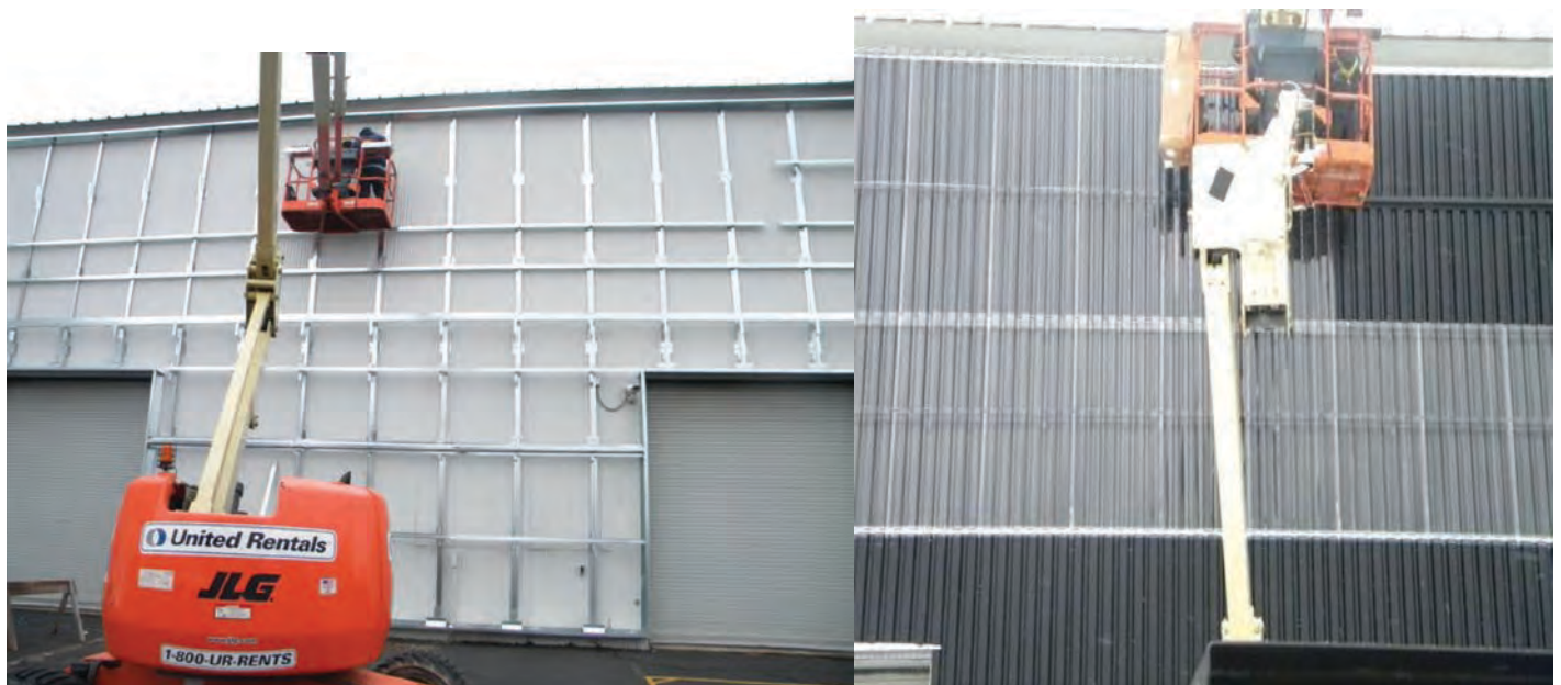
Figure 22-17. Construction of unglazed two-stage SolarWall showing support framing and installation of polycarbonate glazing.
