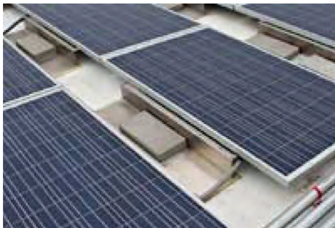
Figure 11-2. Ballasted mounting support structure.
