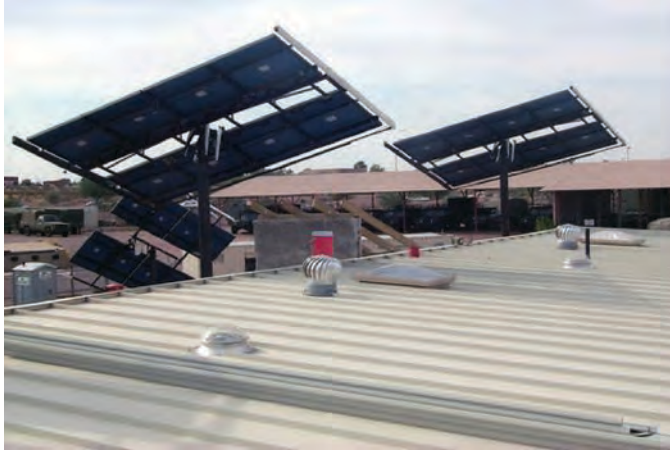
Figure 11-4. Sun-tracking PV systems on the roof of the Arizona National Guard's Eco-Building at Papago Park Military Reservation.
