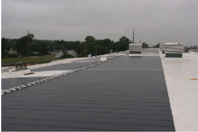
Figure 22-34. TRANSPO roof-integrated thin-film photovoltaic system.
