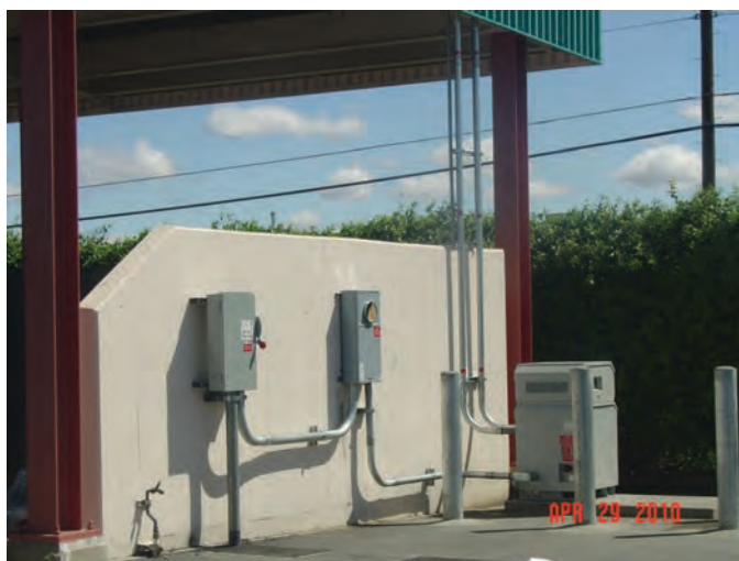
Figure 22-44. Electric interface for the photovoltaic system.
