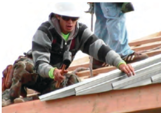
Figure 22-65. Installation of the SSMR panels on roof.
