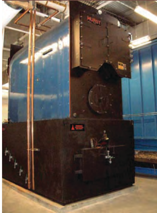
Figure 15-1. Woodchip boiler in Mount Wachusett Community College (MA) biomass plant.
