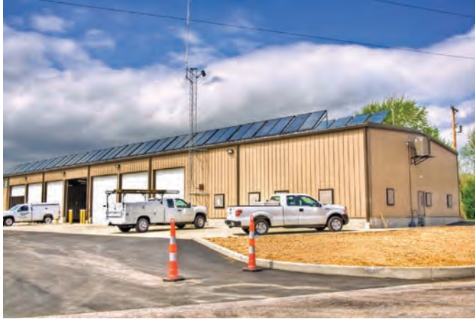
Figure 22-1. Solar air collector array (foreground) and one of the solar water heating system collector arrays (rear row).
