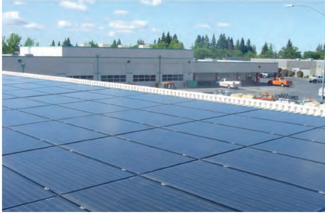
Figure 22-39. A 30-kW photovoltaic system at Sunrise Maintenance Station installed on material storage canopy.
