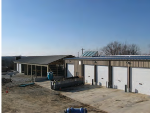
Figure 22-6. Solar collectors for water heating and mounting structure for solar air collectors (foreground).
