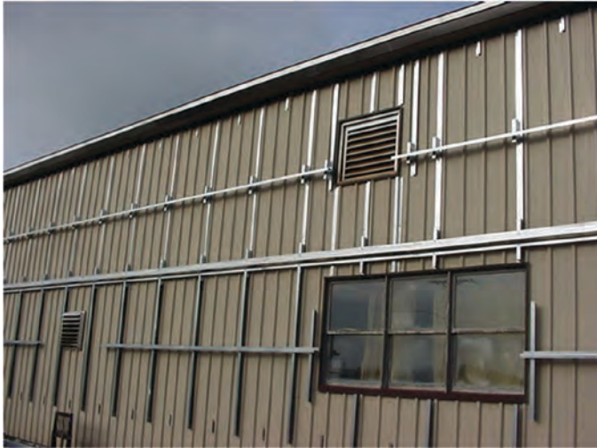
Figure 22-11. Framing structure for SolarWall on Shop Building 91 at Fort Drum.
