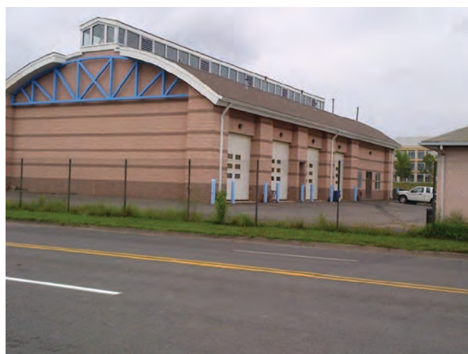
Figure 7-3. Roof monitor on West Ox Road Fairfax, VA, maintenance facility, Virginia Department of Transportation.
