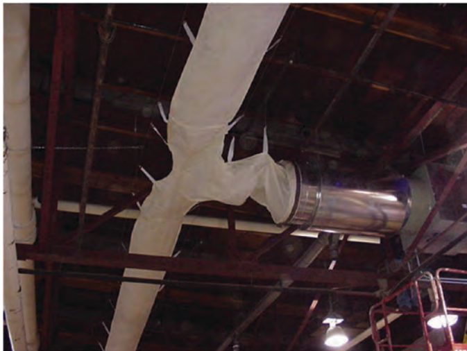
Figure 22-13. Distribution system using flexible ducts with existing system.
