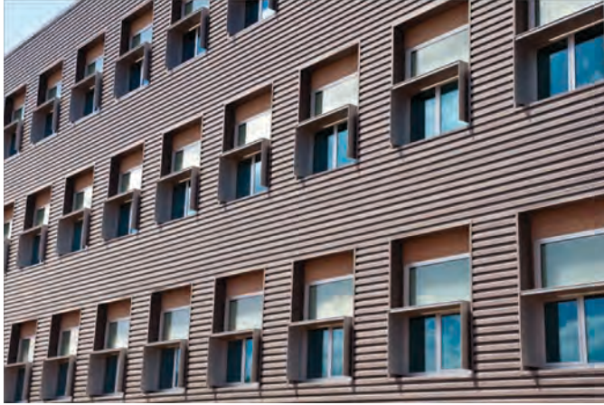
Figure 10-4. Transpired solar collectors on NREL facility.
