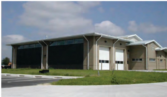
Figure 10-9. Willow Springs, NC, fire hall SolarWall system.
