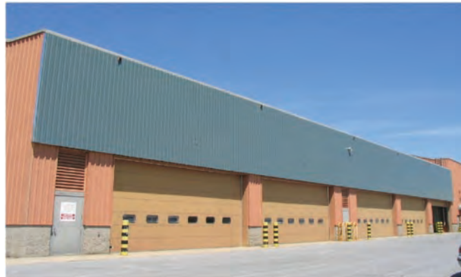
Figure 22-9. Fort Drum Vehicle Maintenance Garage (P-10670) with unglazed transpired collectors (SolarWall) installed above garage doors.
