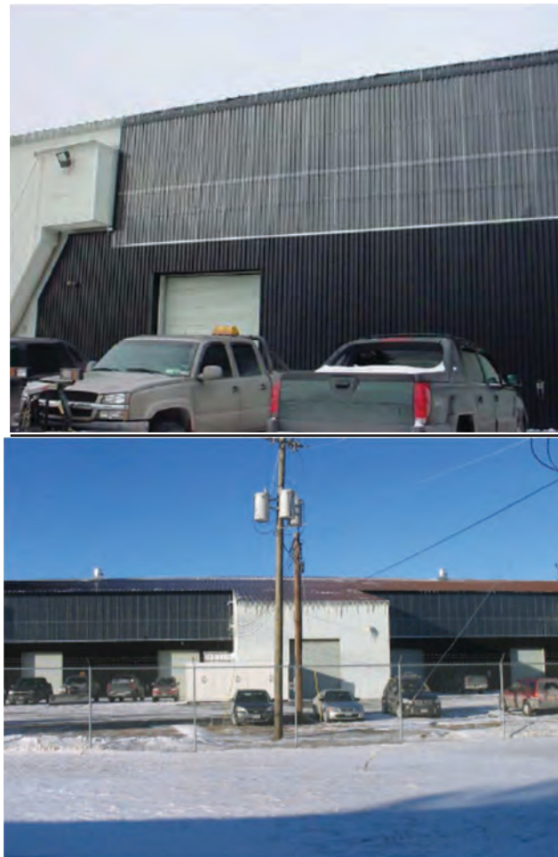
Figure 22-15. Hangar with unglazed transpired collectors (two-stage SolarWall).
