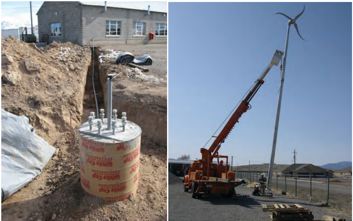
Figure 22-47. Construction of the wind turbine at the Milford Maintenance Station.
