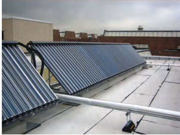
Figure 22-22. Solar collector array and piping layout.
