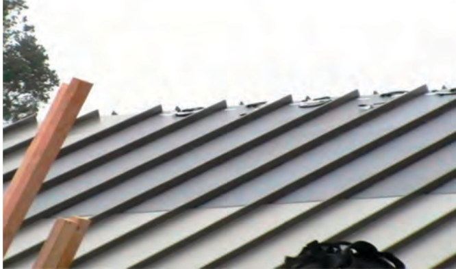
Figure 22-60. Close-up of roof-integrated thin-film photovoltaic system.
