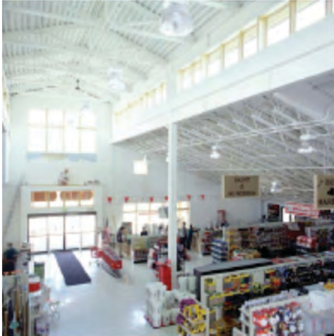
Figure 7-4. Daylighting with clerestory windows at Bighorn Home Improvement Center, Silverthorne, CO.
