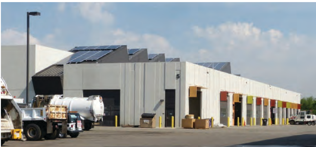
Figure 22-25. Vehicle maintenance building showing PV and shading strategies at doors.
