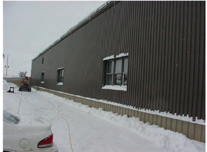
Figure 22-12. SolarWall installed on Shop Building 91 at Fort Drum.
