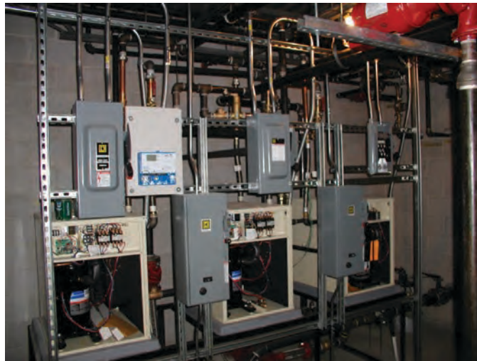
Figure 22-58. Three water-to-water heat pumps supply heat to the radiant heating system in the vehicle bays.
