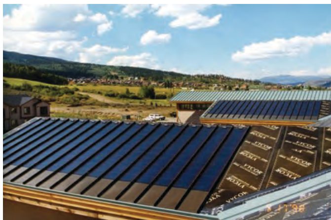
Figure 11-3. Amorphous silicon PV material and metal roofing application—Big Horn Home Improvement Center, Silverthorne, CO.
