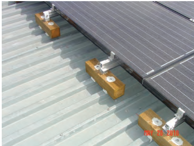
Figure 22-43. Photovoltaic module mounting detail.
