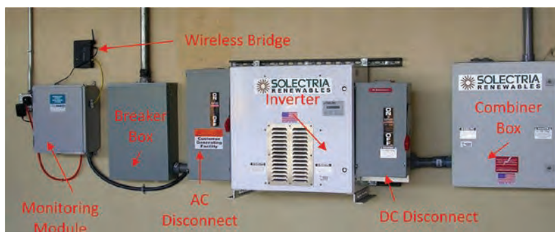
Figure 22-66. Inverter and associated hardware.
