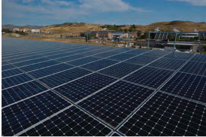
Figure 11-1. Crystalline silicon PV Modules on parking garage at NREL's South Table Mountain facility.
