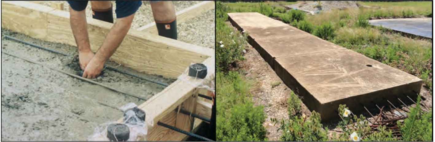
Figure 2.2. Clay lump slab construction.
