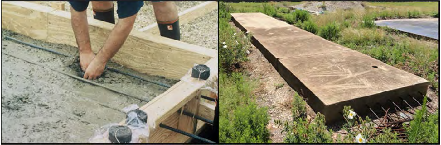
Figure M.7. Clay lump slab construction.
