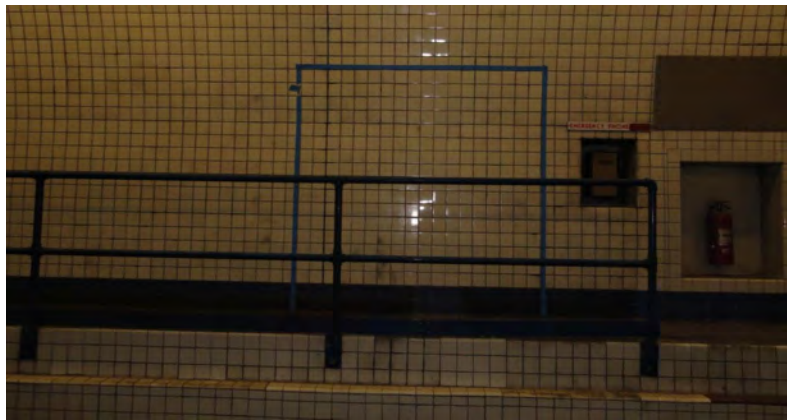
Figure N.31. Image of test site CBBT TILE 10.11-11.
