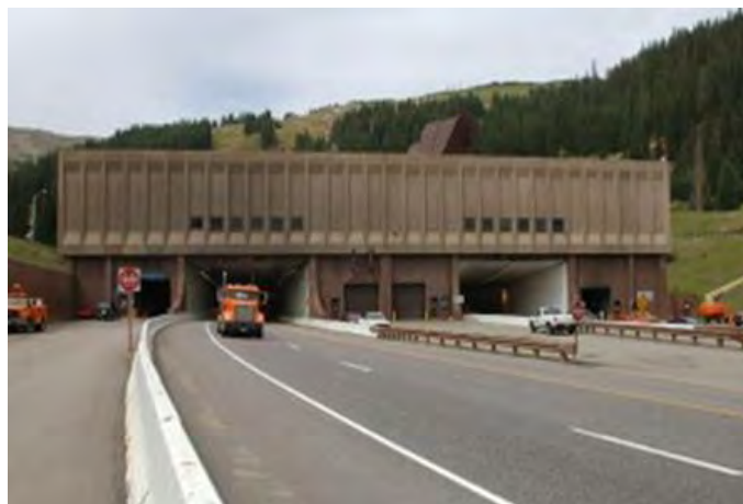
Figure P.2. Outside view of Eisenhower Memorial Tunnel.
