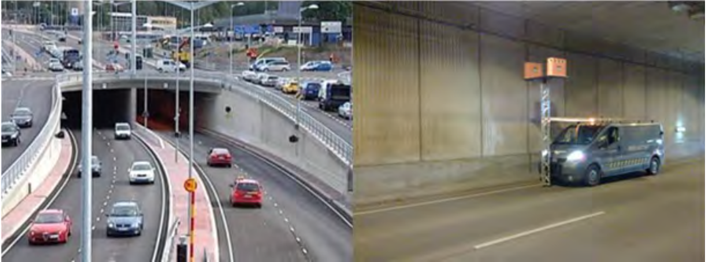
Figure J.10. Hakamäentie Tunnel opening (left) and GPR measurement van in the tunnel (right).
