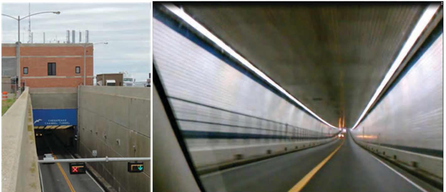
Figure 2.5. Chesapeake Channel Tunnel: entrance (left) and interior view (right).
