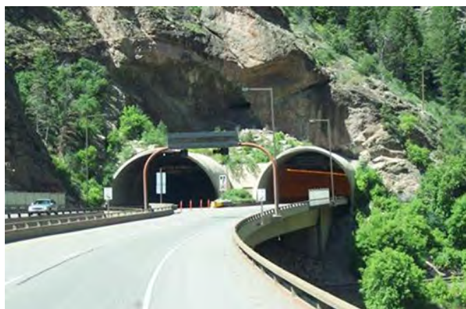
Figure P.3. Outside view of Hanging Lake Tunnel.
