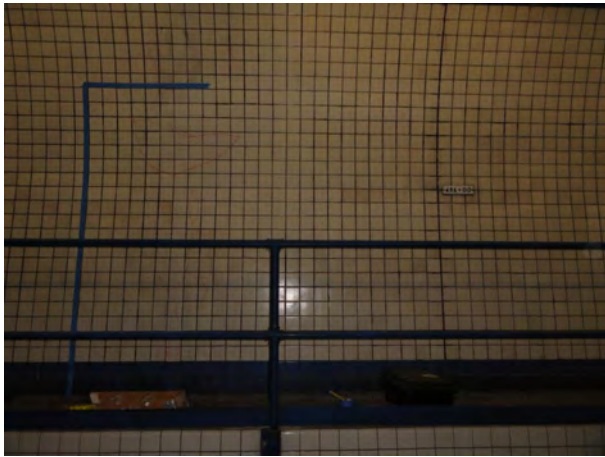
Figure N.33. Image of test site CBBT TILE 10.11-12.
