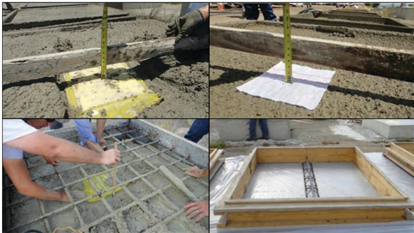
Figure 2.1. Construction of slabs with simulated defects.
