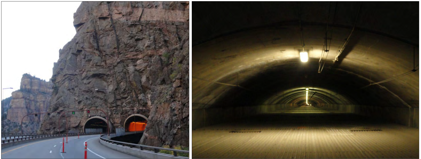
Figure M.36. Hanging Lake Tunnel: exterior view (left) and interior plenum view (right).
