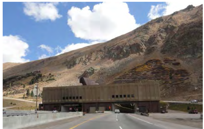
Figure M.29. Eisenhower Memorial Tunnel, Colorado.
