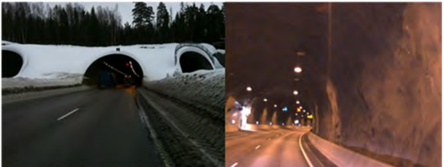
Figure J.12. Exterior and interior views of Vuosaari test tunnel. The A-tunnel opening is on the mainland, the railway tunnel is to its right, and the B-tunnel is on the left.
