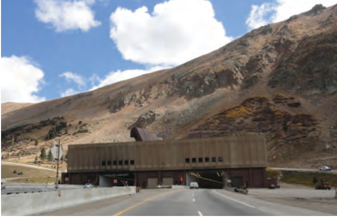
Figure 2.6. Eisenhower Memorial Tunnel, Colorado.
