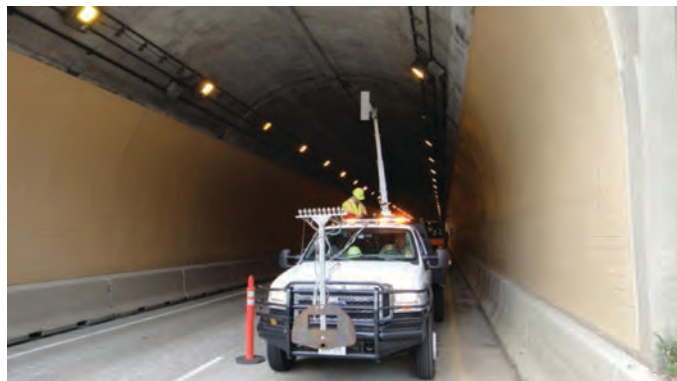
Figure 2.9. TTI air-coupled GPR system collecting data in No Name Tunnel.
