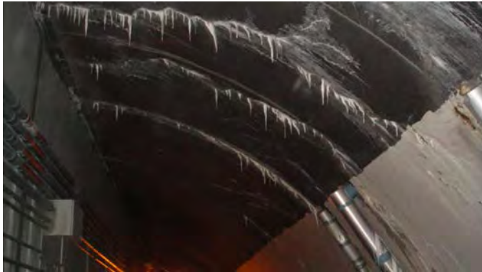
Figure L.17. Visual image of the top of the Eisenhower Memorial Tunnel.
