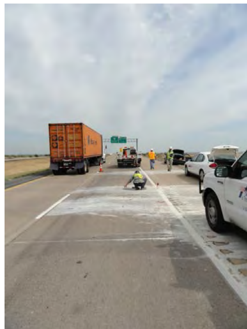
Figure M.21. I-20 in Fort Worth, Texas.
