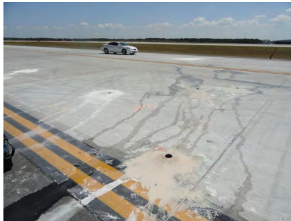
Figure N.53. Image of test site IAH 6.9-1.
