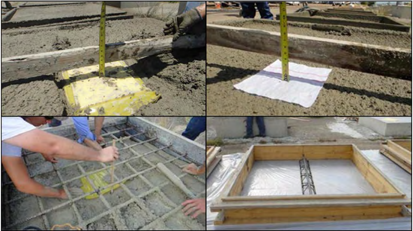
Figure M.3. Construction of slabs with simulated defects.
