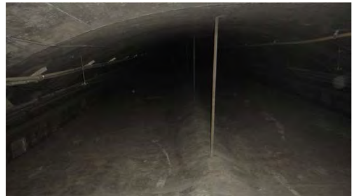
Figure L.6. Visual image of the top of the Chesapeake Channel Tunnel.
