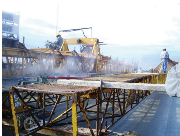
FIGURE 10 Fogging equipment is used to control evaporation rates [Photo courtesy of the University of Kansas Transportation Research Institute].
