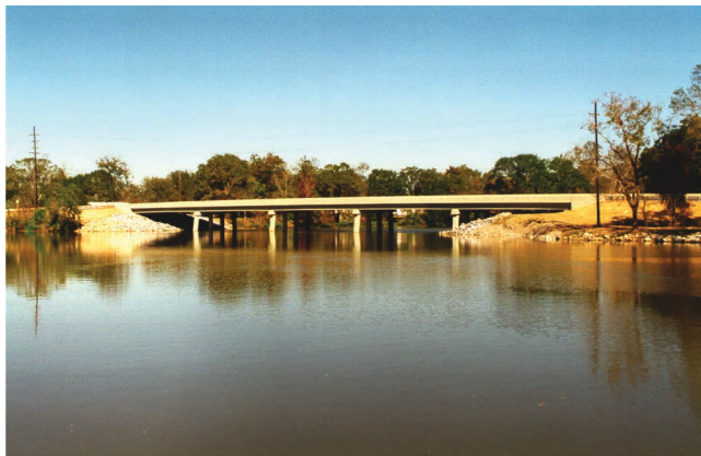
FIGURE 14 High performance concrete was used in all components of the Charenton Canal Bridge in Louisiana [Photo courtesy of Louisiana Department of Transportation, Bridge and Structural Design Section].
