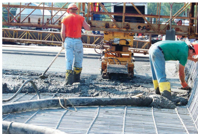
FIGURE 15 Placement of Class HP concrete [Photo courtesy of NYSDOT].
