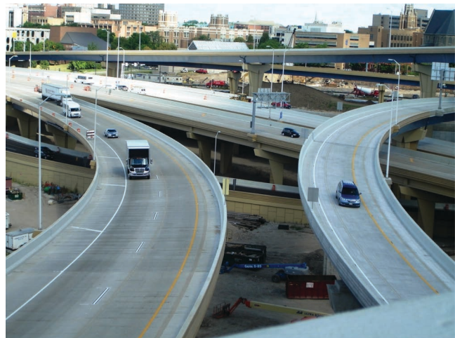
FIGURE 16 The Marquette Interchange in Milwaukee, Wisconsin, used the second generation of HPC specifications [Photo courtesy of Tony Straseske, Wisconsin Department of Transportation].
