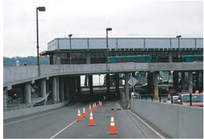
FIGURE 24 Elevated busway serves transit center on land-side of Bremerton Transportation Center ( Courtesy: Nelson\Nygaard Consulting Associates ).
