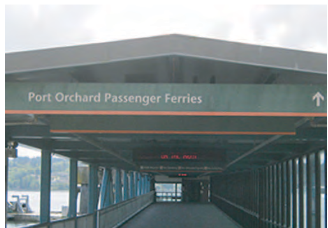
FIGURE 25 Covered walkway with signage directs passengers to Kitsap Foot Ferry ( Courtesy: Hayward Seymore ).
