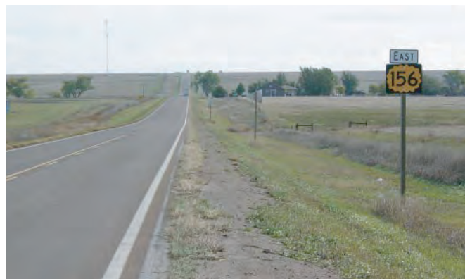
Before improvements were made along K-156, a sloping dirt shoulder didn't allow motorists adequate room to pull off of the highway.
