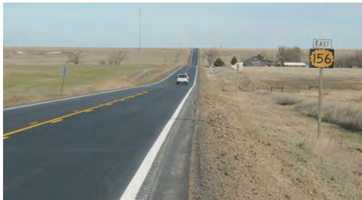
After improvements along K-156 in Hodgeman County, the benefits include a wider shoulder, rumble strips and a gentler side slope.
