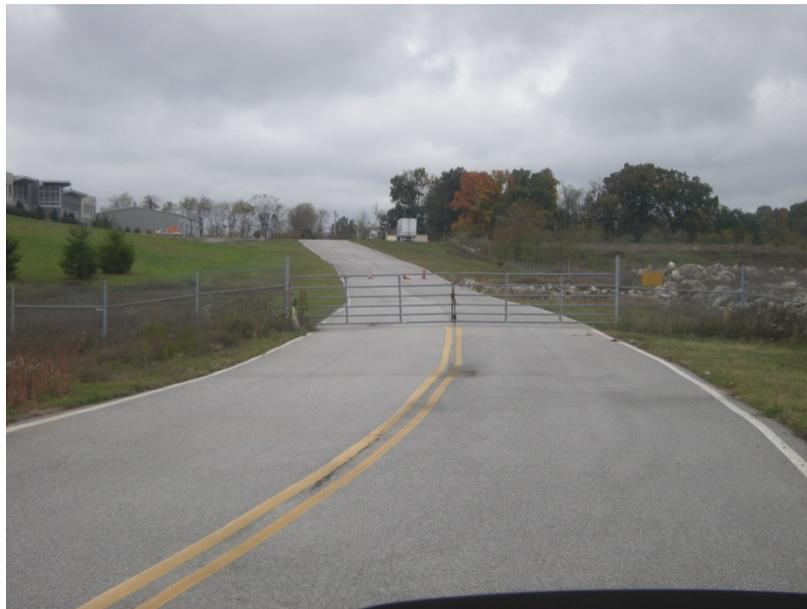
*Figure 23. Secondary sag vertical curve on the Smart Road.*
