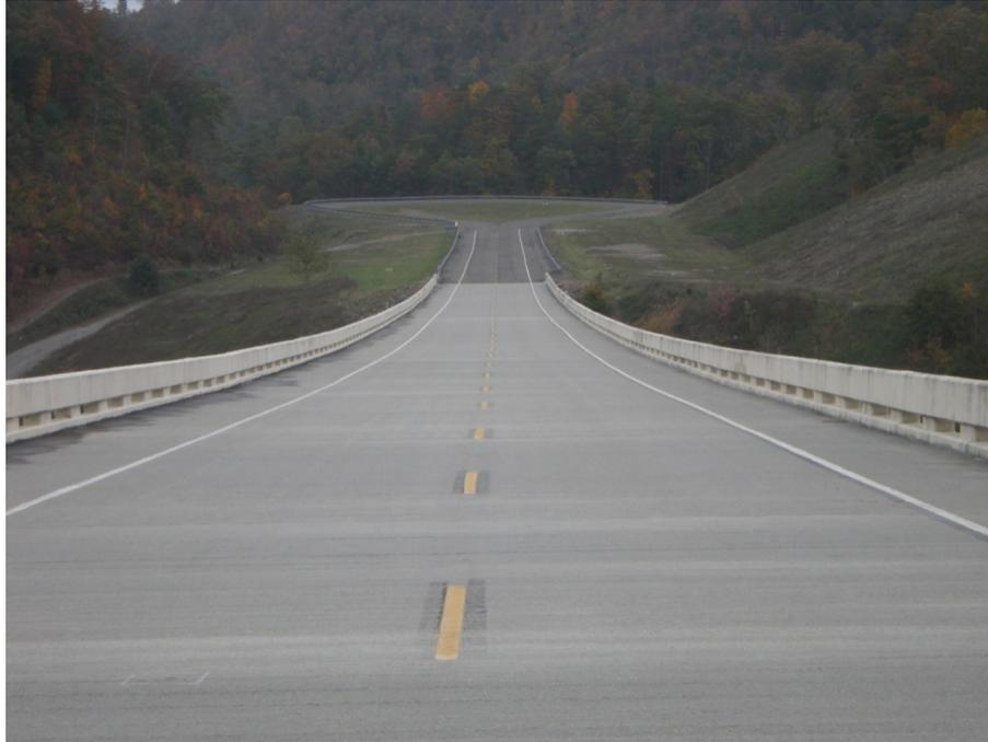
*Figure 22. Primary sag vertical curve on the Smart Road.*
