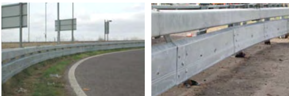
FIGURE 2 The Cloverleaf Junction following the installation of the MPS.
