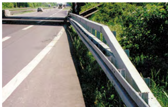
FIGURE 3 Higher barrier to protect gantries and bridge piers.
