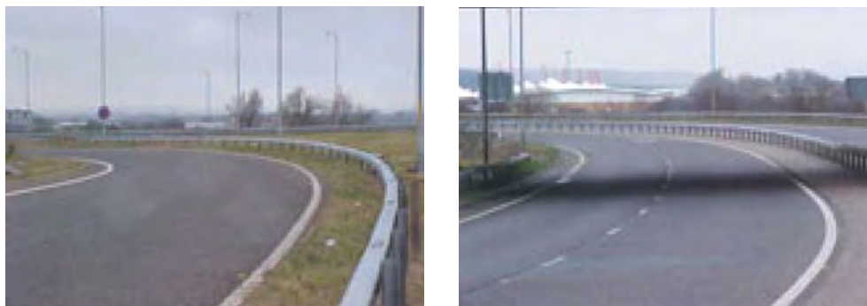
FIGURE 1 The Cloverleaf Junction before the installation of the MPS.
