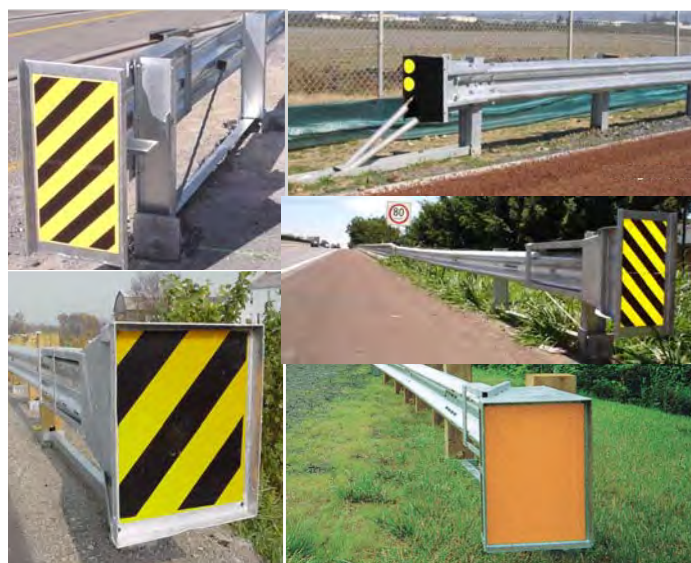
FIGURE 5 Examples of crashworthy terminals.
