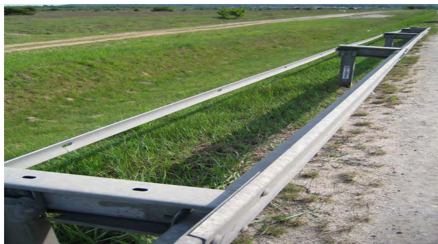
FIGURE 6 Inappropriate post spacings.
