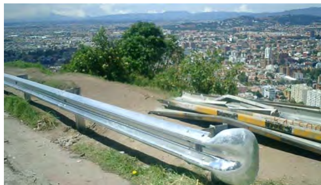
FIGURE 6 Spoon terminal in South America.
