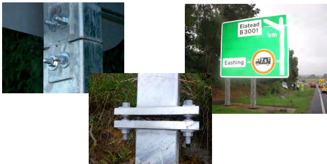
FIGURE 6 Passively safe support structures (la Torre, 2011).
