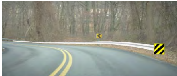
FIGURE 10 Potential solution by extending the guardrail.
