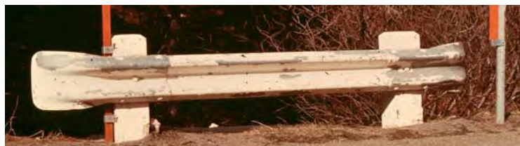
FIGURE 1 Typical fishtail or spoon terminal.
