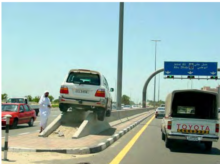
FIGURE 7 Turned-down concrete terminal in Middle East.
