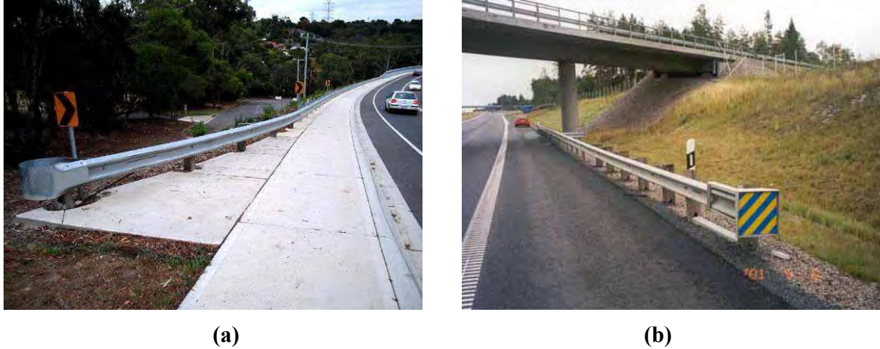
FIGURE 2 Crashworthy barrier terminals: (a) Tasmania (2004) and (b) Riser (2006).
