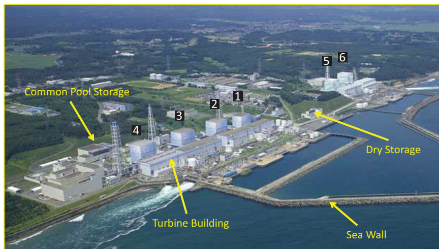
FIGURE 1.2 Oblique aerial photo of the Fukushima Daiichi Nuclear Power Station prior to the March 11, 2011, Great East Japan Earthquake and tsunami. Locations of reactor units are indicated by their numbers (i.e., Units 1-6). Locations of the turbine buildings, seawall, and common spent fuel storage (pool and dry) are also indicated. SOURCE: Courtesy of TEPCO.
