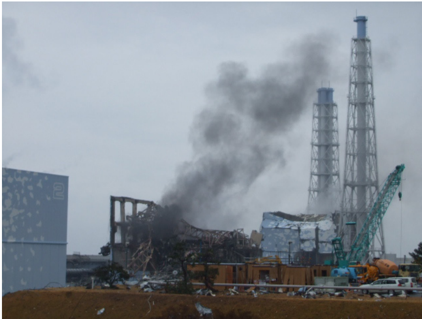
FIGURE 3.9 March 21, 2011, photo of damaged Unit 3 (middle) and Unit 4 (right) reactor buildings. Unit 2 is shown on the left margin of the photo. SOURCE: Courtesy of TEPCO ( http://photo.tepco.co.jp/en/date/2011/201103-e/110321-01e.html ).
