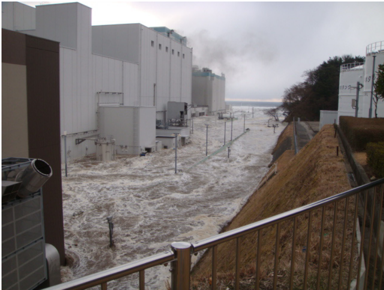
FIGURE 3.11 Photo showing flooding of the Fukushima Daini plant adjacent to Unit 1 during the March 11, 2011, tsunami. Flooding depth was between 2-3 m. SOURCE: Courtesy of TEPCO ( http://photo.tepco.co.jp/library/110411_3/110412_2f_tsunami_6.jpg ).
