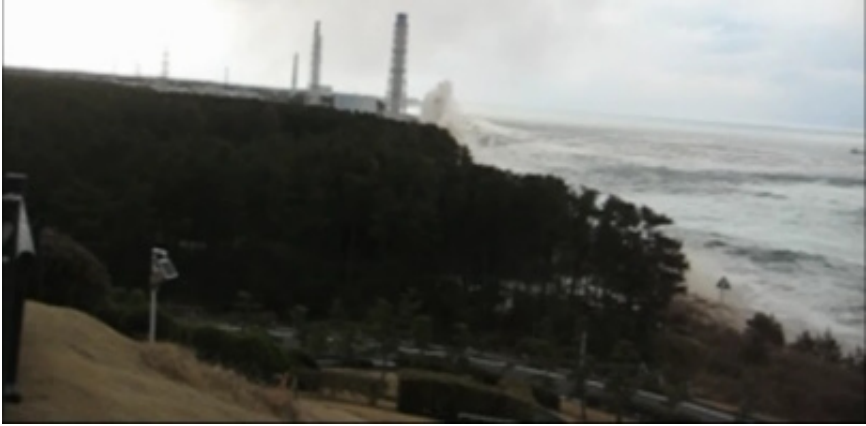
FIGURE 3.7 Photo taken looking north toward the Fukushima Daiichi plant on March 11, 2011. The photo shows the tsunami wave as it strikes the seaward side of the plant. Flooding can also be seen in the foreground of the photo. SOURCE: Courtesy of TEPCO ( http://photo.tepco.co.jp/library/110409/110409_1f_tsunami_1t.jpg ).
