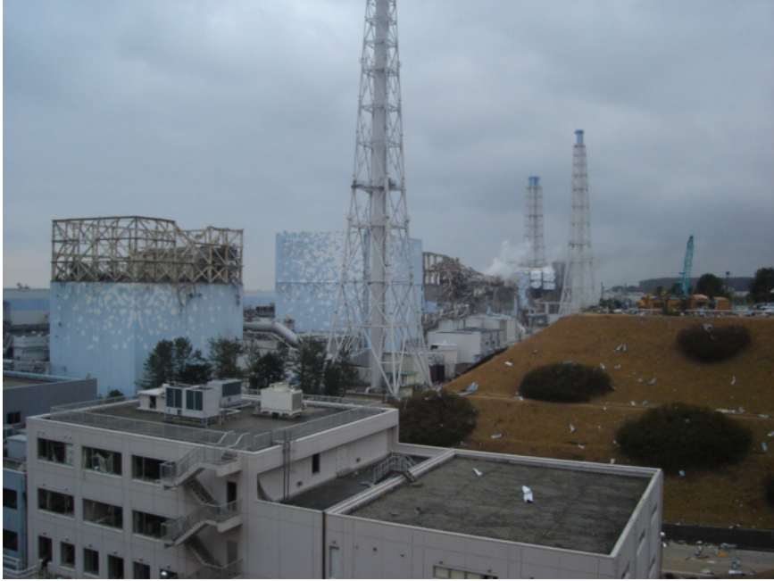
FIGURE 1.3 March 16, 2011, photo of the Fukushima Daiichi Nuclear Power Station showing damaged Units 1 (foreground), 3, and 4 reactor buildings. SOURCE: Courtesy of TEPCO ( http://photo.tepco.co.jp/library/110316/110316_1f_chijou_2.jpg ).
