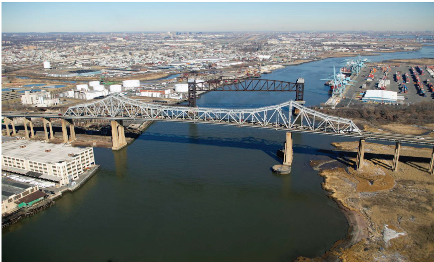
FIGURE 2 Existing Goethals Bridge (Foreground)
