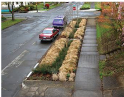
Behind the curb swale / basin
