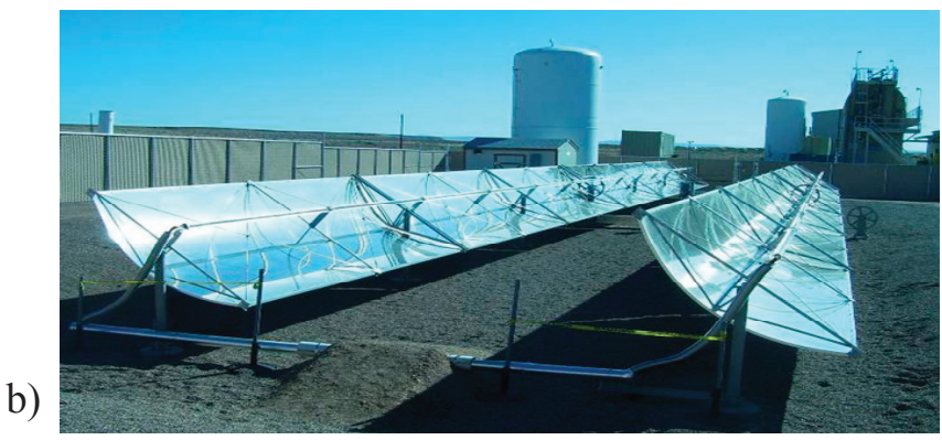
FIGURE 4-5 The Tuba City site is located in northeastern Arizona on the western edge of the Navajo Nation (a). A solar voltaic field provides part of power for ground water treatment system and is tied to the local grid (b). SOURCE: Geiser 2014.
