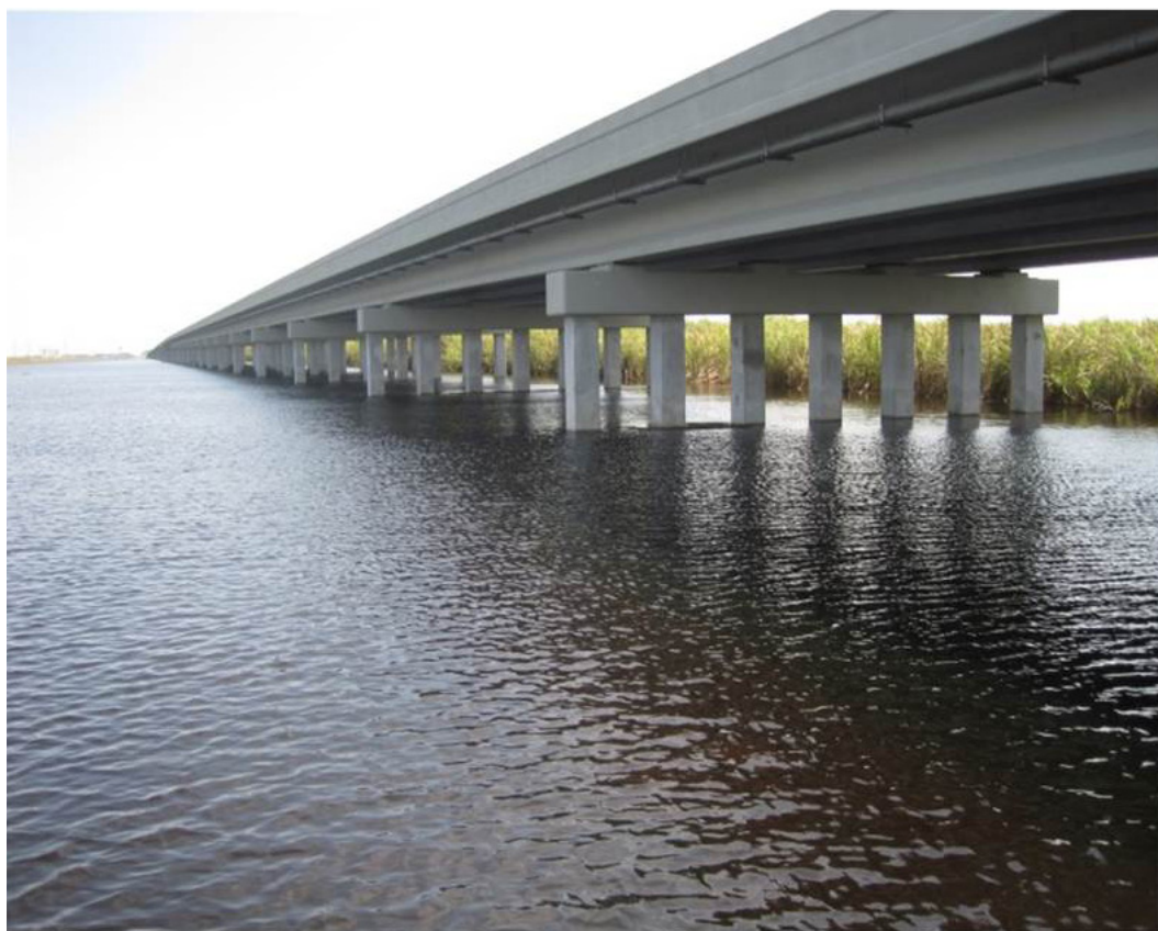
FIGURE 4-22 The newly constructed 1-Mile Tamiami Trail bridge, showing conveyance area beneath the newly elevated highway.
