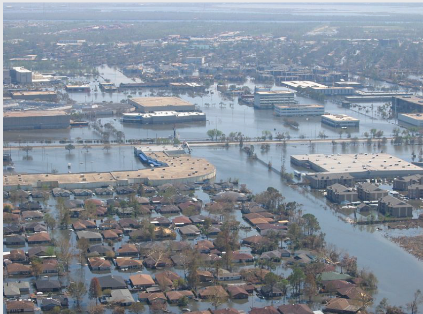
FIGURE 1-4-1 Flooding of New Orleans after Hurricane Katrina.
