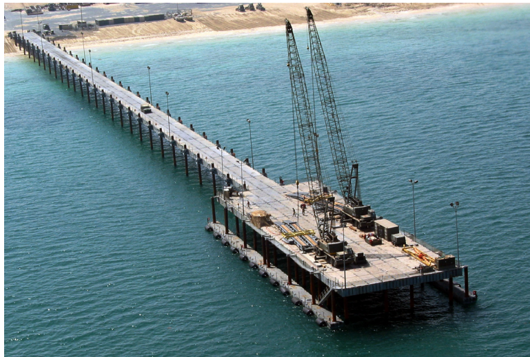
FIGURE 4-11 ELCAS-M in place. SOURCE: U.S. Navy photo by Journalist 1st Class Joseph Krypel. [Public domain], via Wikimedia Commons, http://commons.wikimedia.org/wiki/File:US_Navy_030426-N-1050K-052_The_U.S._Navy's_Elevated_Causeway_System-Modular_(ELCAS-M)_stands_completed_at_Camp_Patriot.jpg .
