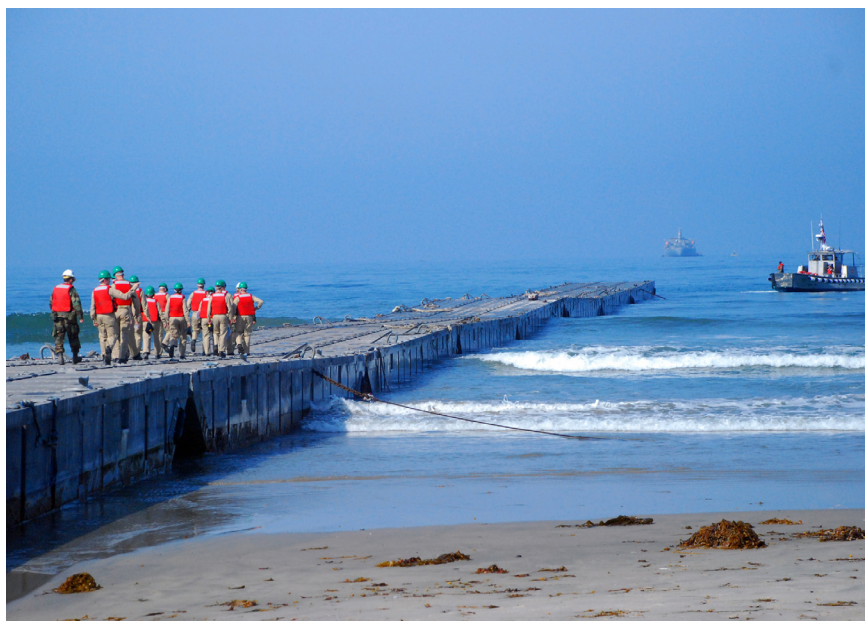
FIGURE 4-10 Deployed JLOTS causeway segments. SOURCE: U.S. Navy photo by Mass Communication Specialist 3rd Class Brian Morales [public domain], via Wikimedia Commons, http://commons.wikimedia.org/wiki/, File: US_Navy_080715-N-4973M-028_Midshipmen_walk_along_the_Joint_Logistics_Over-The-Shore_(JLOTS)_Admin_Pier,_an_800-foot_long,_small-craft_pier.jpg .
