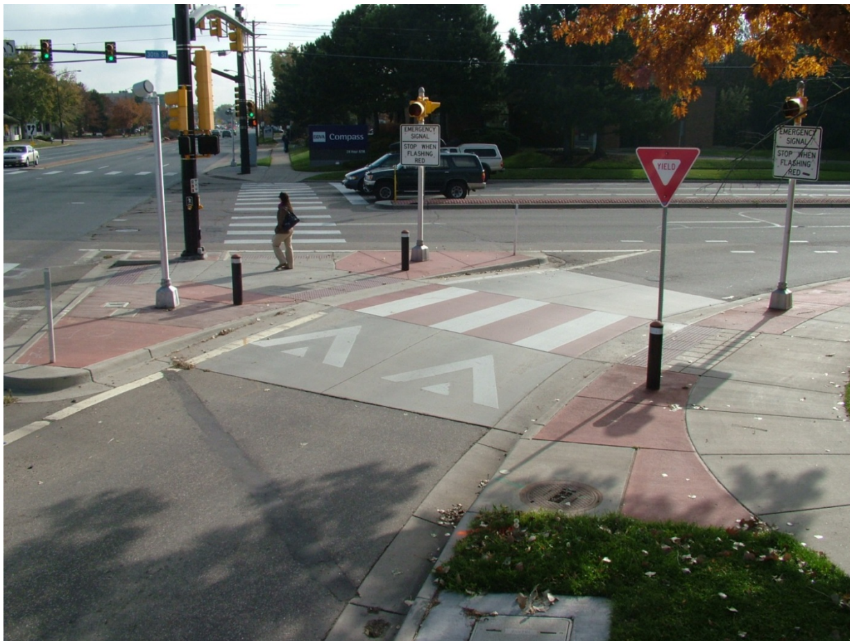
Figure 14. Raised Crosswalk at Channelized Right-Turn Lane in Boulder, Colorado
