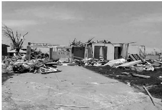
Figure 7.4. Debris generated from a tornado. (Source: FEMA)
