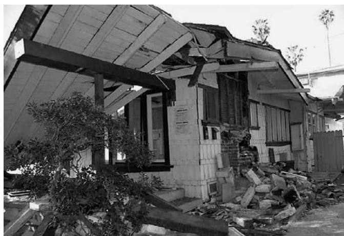
Figure 7.6. Debris generated from an earthquake. (Source: FEMA)
