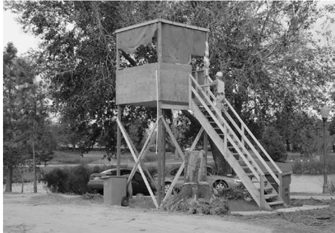
Figure 10.3. Wooden structure inspection tower. (Source: FEMA)
