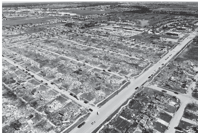
Figure 3.1. Damage to residential development by tornado. (Source: FEMA)
