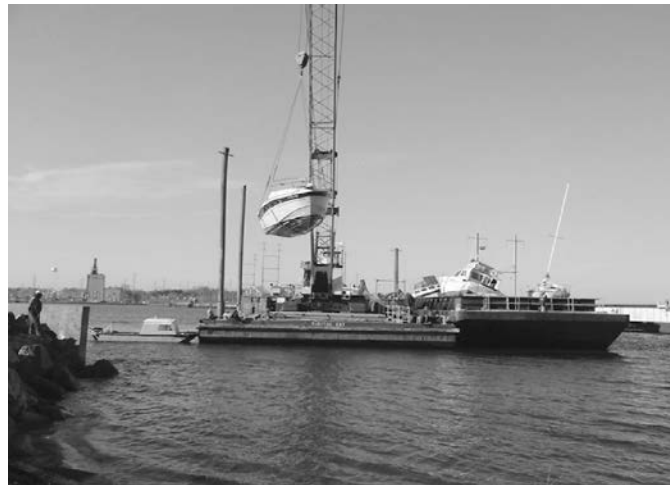
Figure 7.12. Marine debris removal by point pickup method. Hurricane Sandy, New Jersey. (Source: Ali Velasco)
