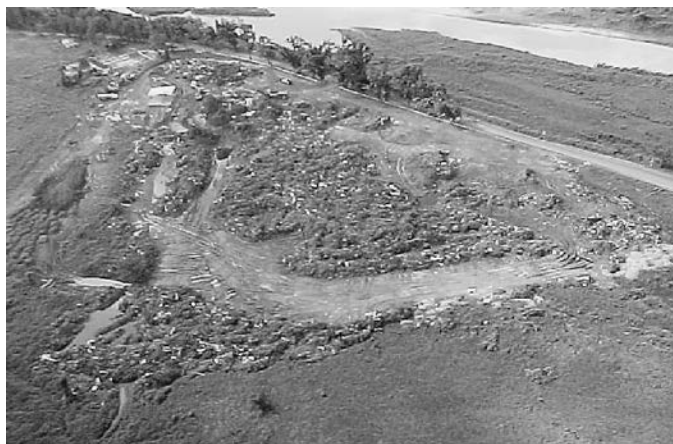
Figure 13.1. Located near a body of water and in a wetlands, this DMS does not meet environmental criteria for site selection. (Source: FEMA)
