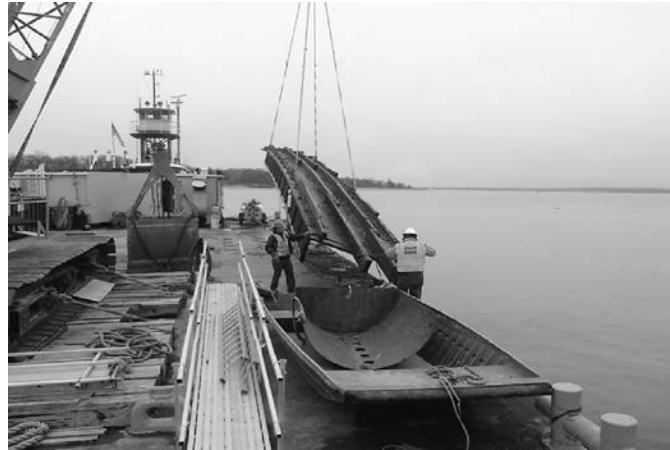
Figure 7.11. Marine debris removal by point pickup method. Hurricane Sandy, New Jersey. (Source: Ali Velasco)
