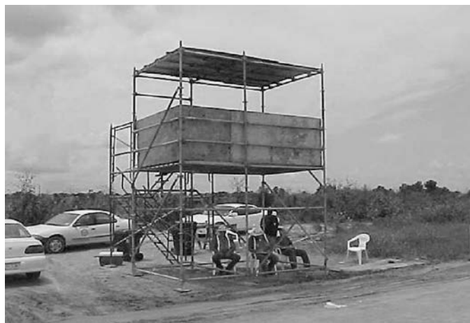
Figure 10.6. Inspection tower at landfill. Debris monitors on site, making capacity calls. (Source: FEMA)
