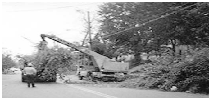
Figure 7.2. Crew opening a blocked lane into a residential area. The debris that is piled up on the road is being hauled. (Source: FEMA)
