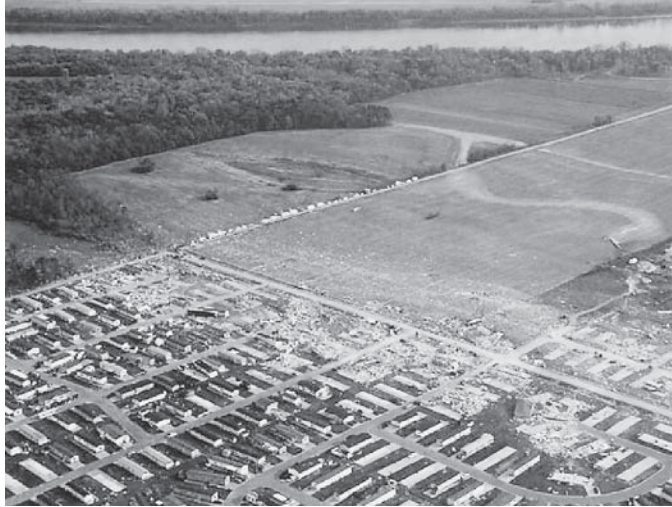
Figure 3.2. Damage to mobile home park 2005 Evansville area tornado. [Source: National Oceanic and Atmospheric Administration (NOAA)]
