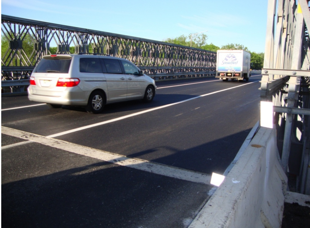
FIGURE 7 Rt. 80 ACROW bridge with New Jersey DOT's BDWSC asphalt overlay.
