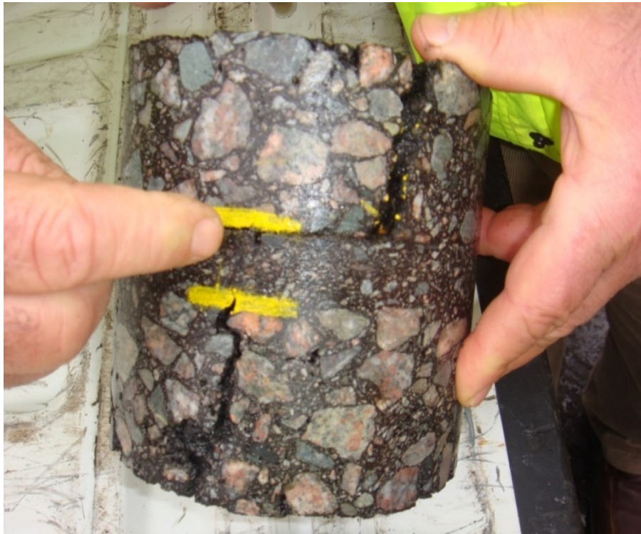
FIGURE 4 Cracking above and below a highly fatigue resistant mixture.
