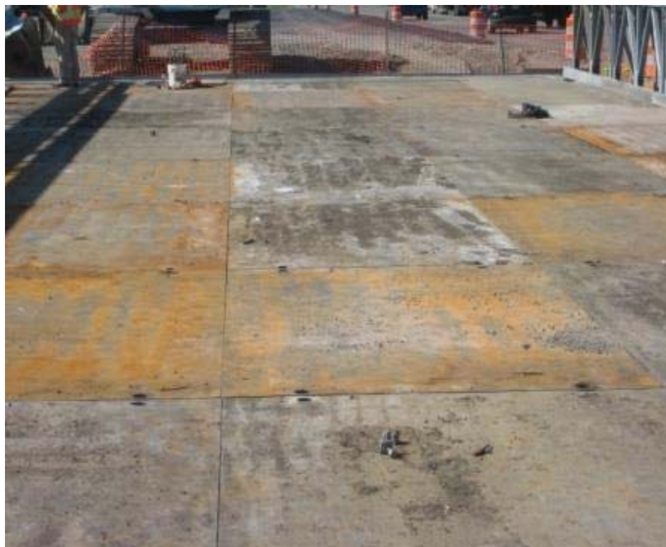
FIGURE 5 Steel deck ACROW bridge on Rt. 80 in New Jersey.
