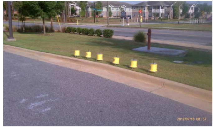
Figure 4.10. Sensor line between clean out and manhole.
