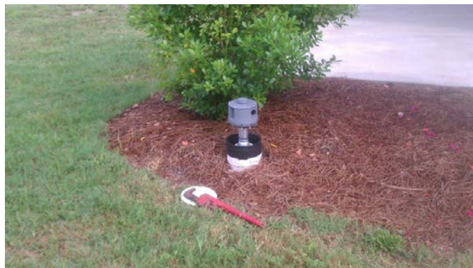
Figure 4.7. Signal injection speaker in clean out near 28th Street and Talbotton.
