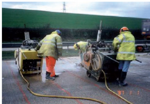
Figure 2.7. Sawing concrete slabs. Source: Jordan et al., 2008.
