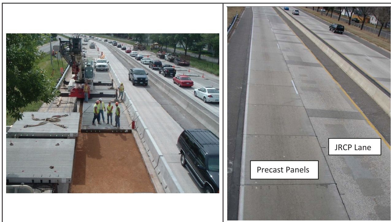
Figure 6.5. Precast section, Minnesota TH-62.
