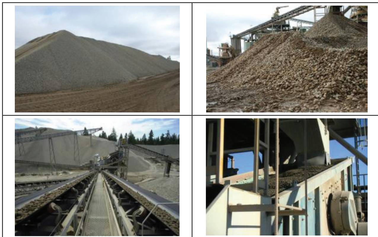
Figure 3.14. Aggregate processing, which includes stockpiles, conveyors, and screening. Photos: Joe Mahoney.
