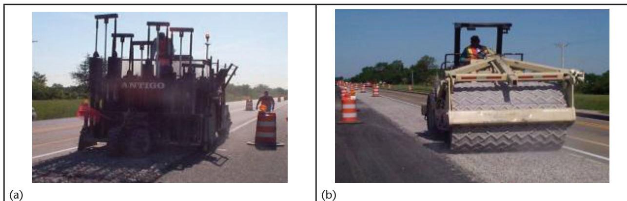
Figure 2.10. (a) Multihead breaker. (b) Grid roller. Source: Baladi et al., 2000.
