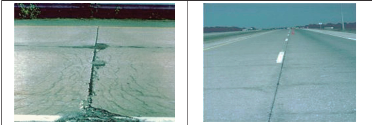
Figure 3.15. D-cracking.
