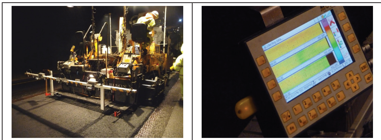
Figure 2.32. Pave-IR thermal imaging system.
