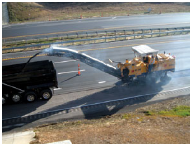
Figure 2.1. Typical milling operation of existing HMA layer. Source: WSDOT, 2010.
