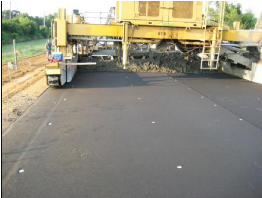
Figure 3.25. Placement of nonwoven fabric as an interlayer. Source: Tayabji et al., 2009.
