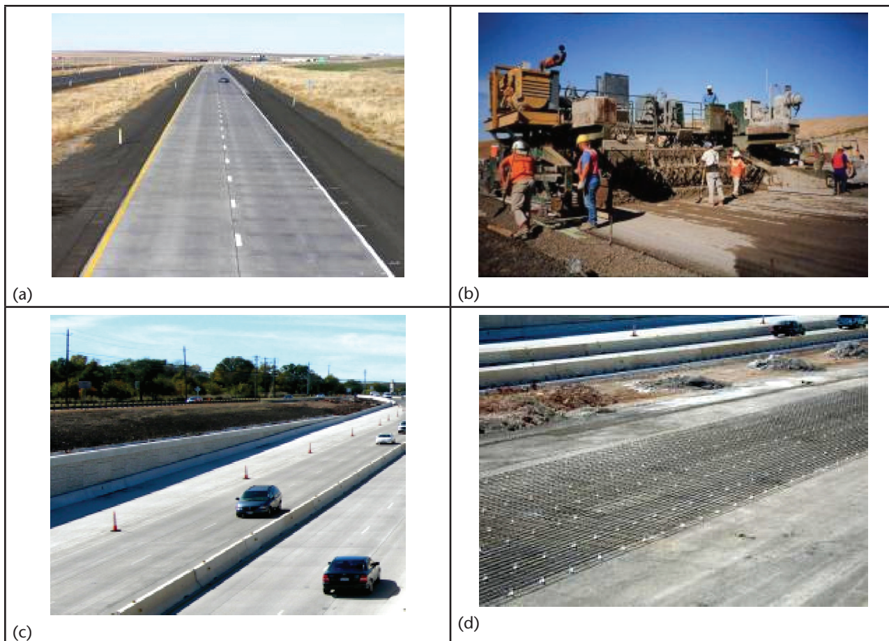
Figure 3.1. Completed and under-construction JPCP and CRCP. (a) and (b) JPCP constructed on HMA base. (c) and (d) CRCP constructed on HMA base. Photos: Joe Mahoney.
