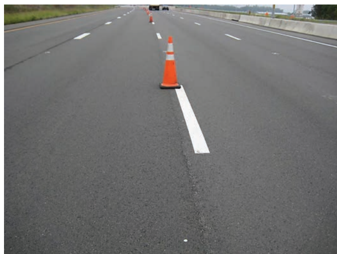
Figure 1.59. WMA and HMA sections in Centreville, Virginia, at 15-month inspection.
