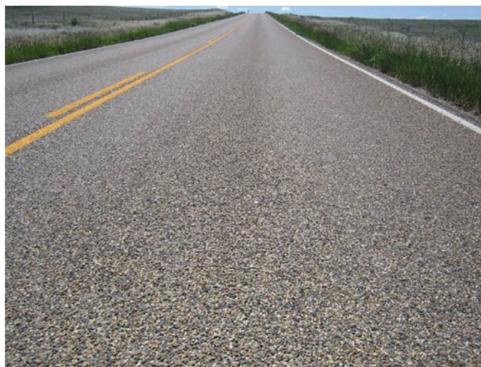
Figure 1.77. HMA control section at 22-month inspection, Baker, Montana.
