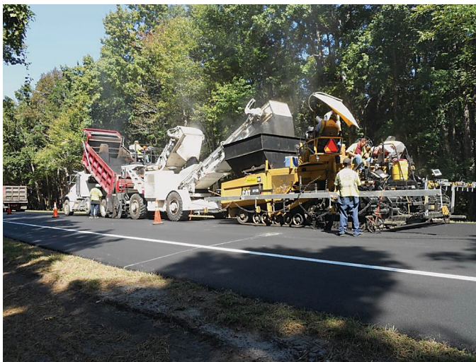
Figure 1.96. MTV transferring mix into the paver in Jefferson County, Florida.
