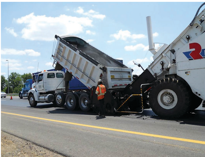
Figure 1.55. Truck dumping into MTV in Centreville, Virginia.
