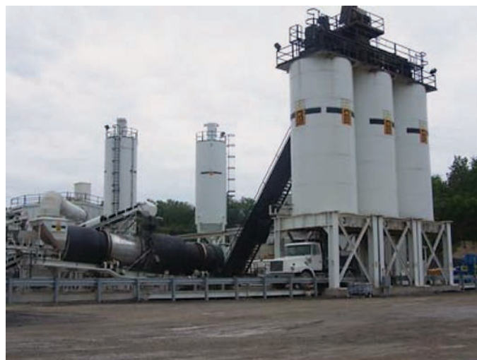
Figure 1.13. CMI counter-flow drum plant in St. Louis, Missouri (23).
