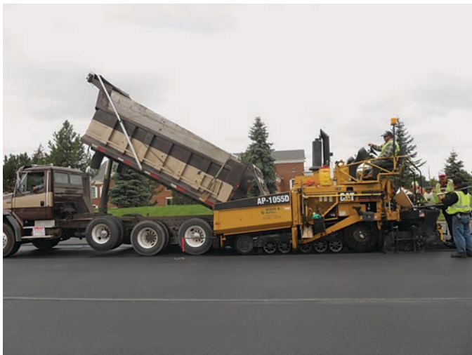
Figure 1.85. Truck dumping into Caterpillar AP-1055D paver.
