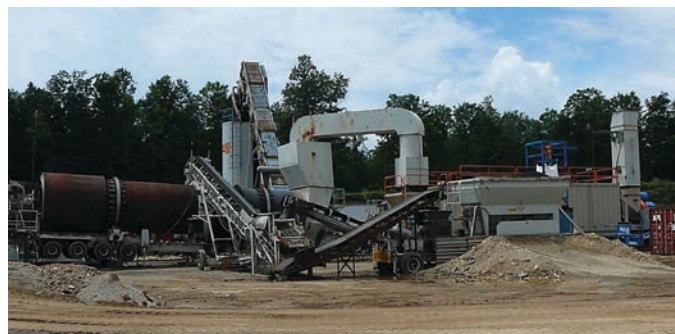
Figure 1.64. Parallel-flow portable drum plant in Rapid River, Michigan.
