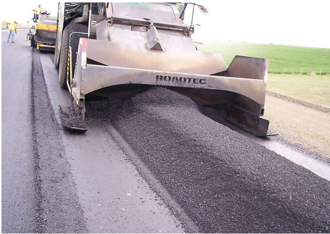
Figure 1.44. Material transfer device and windrow in Walla Walla, Washington.
