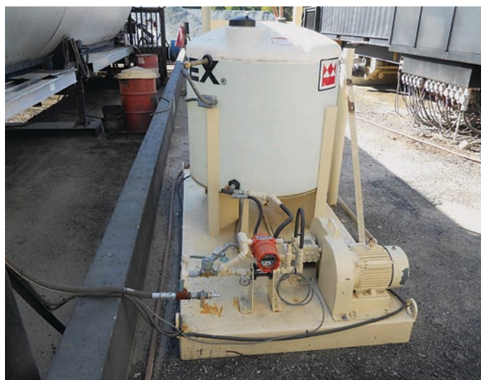
Figure 1.93. Terex WMA system used in Jefferson County, Florida.
