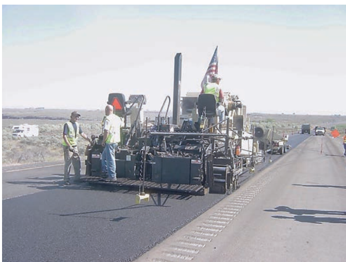
Figure 1.37. Paver spreading mix in George, Washington.
