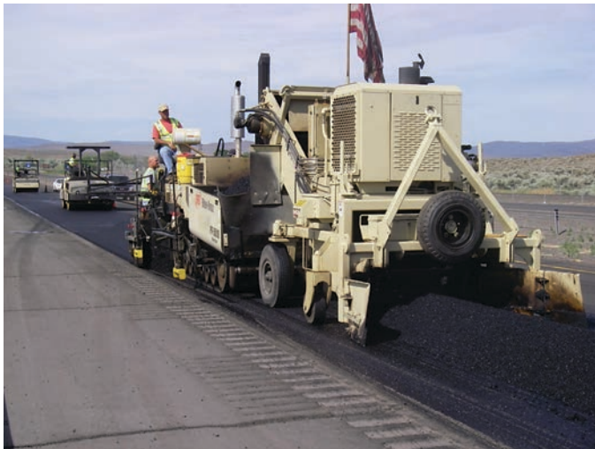
Figure 1.36. Windrow elevator transferring mix to Paver in George, Washington.
