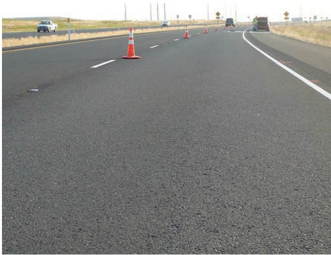
Figure 1.50. Surface texture in Walla Walla, Washington, at 27-month inspection.
