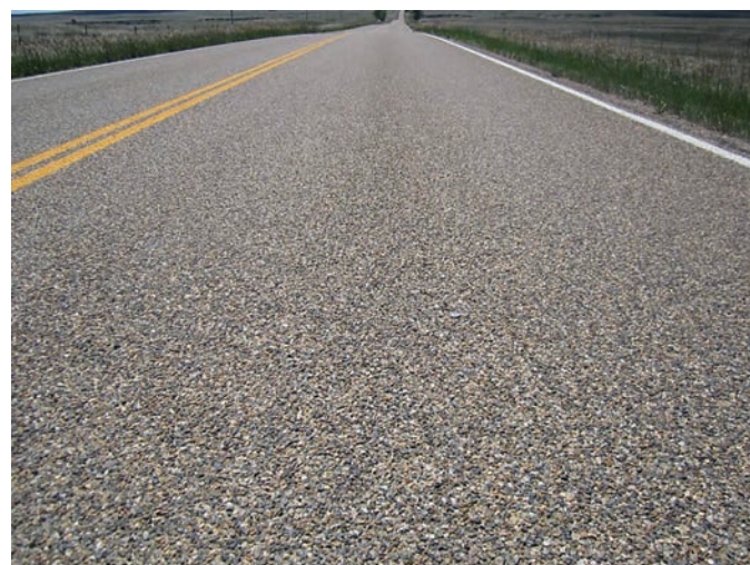
Figure 1.78. Evotherm DAT section at 22-month inspection, Baker, Montana.
