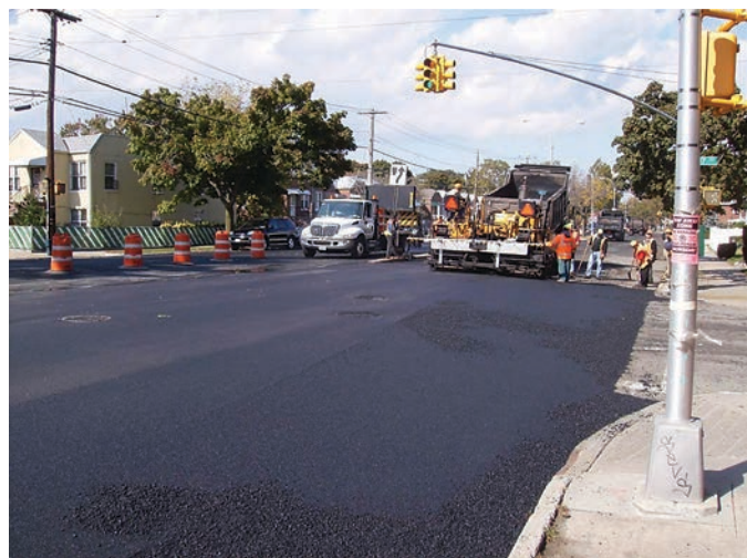
Figure 1.114. Typical hand work in urban paving project.
