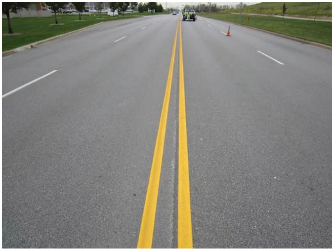
Figure 1.88. Foam, Evotherm, Wax, and HMA sections, respectively, in Munster, Indiana.
