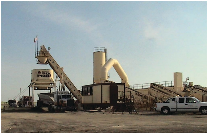
Figure 1.29. Portable asphalt plant used for Graham, Texas, project.
