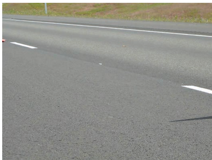
Figure 1.47. WMA (foreground) and HMA (background) sections in Walla Walla, Washington, at 13-month inspection.
