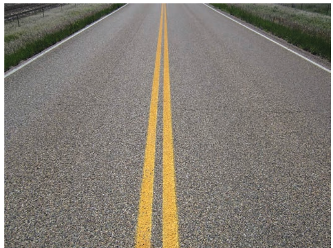
Figure 1.76. Low-severity transverse cracking at 22-month inspection, Baker, Montana.
