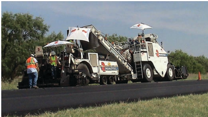
Figure 1.32. Material transfer device and paver used for Graham, Texas, project.
