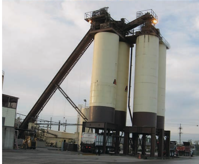
Figure 1.83. Counter-flow drum plant in Griffith, Indiana.
