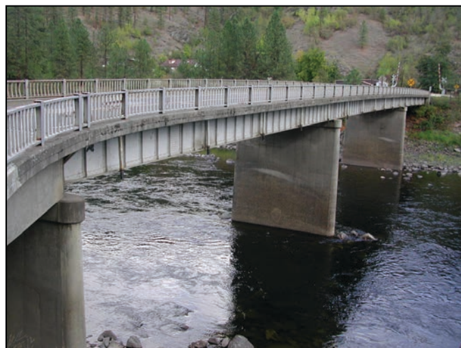
Figure F2. Elevation view of Example Bridge 2.
