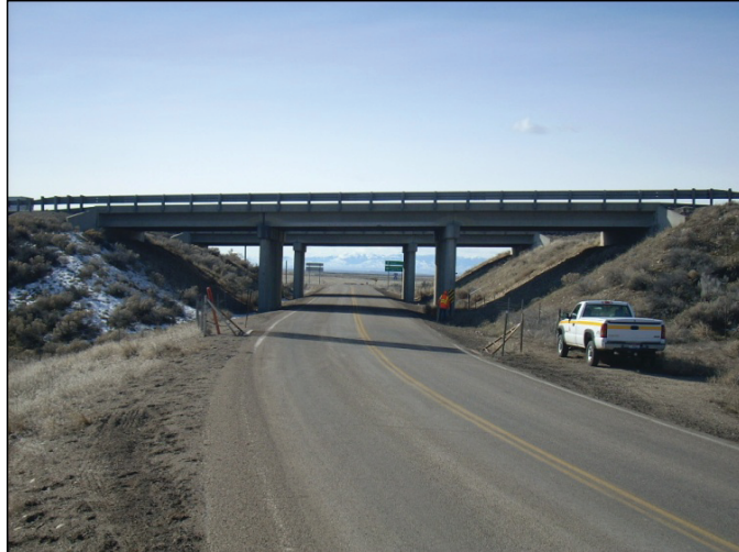
Figure F3. Elevation view of Example Bridge 3.
