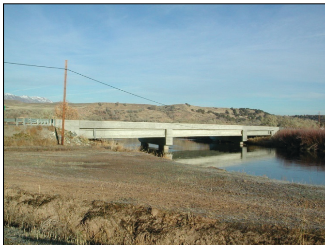
Figure F1. Elevation view of Example Bridge 1.
