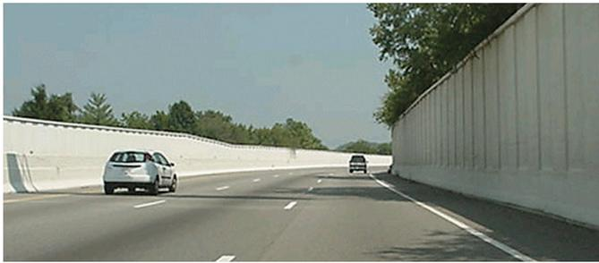
Figure 55. Highway with parallel noise barriers on opposite sides of the road.<sup>58</sup>
