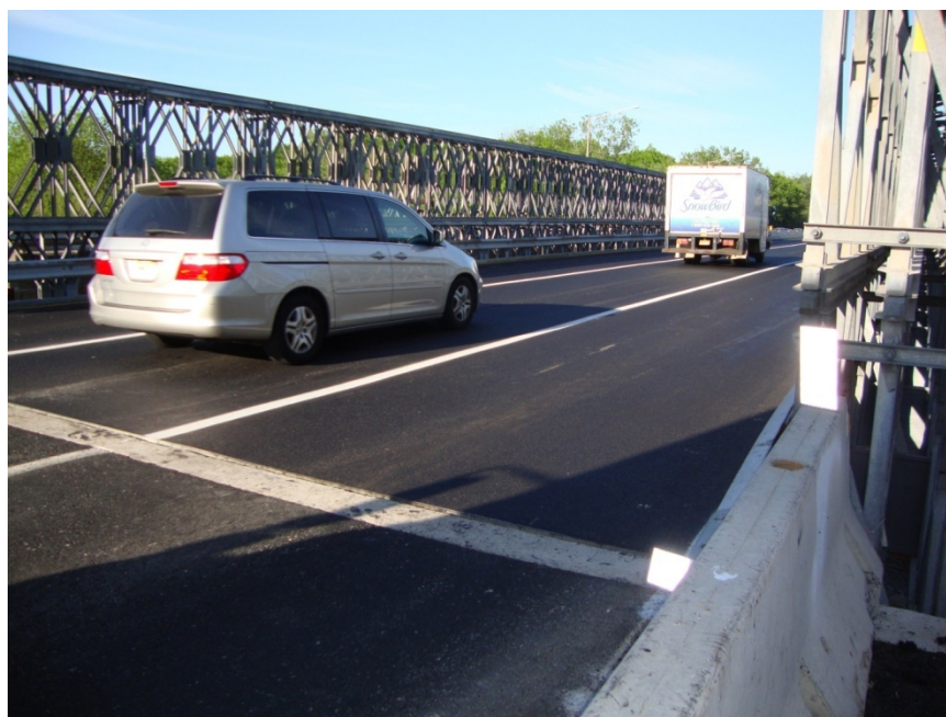
FIGURE 7 Route 80 ACROW Bridge with New Jersey DOT's BDWSC asphalt overlay.
