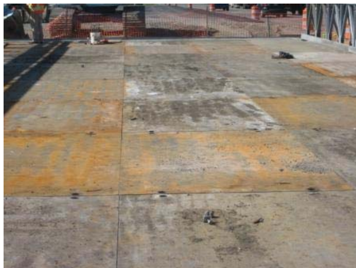
FIGURE 5 Steel deck ACROW bridge on Route 80 in New Jersey.
