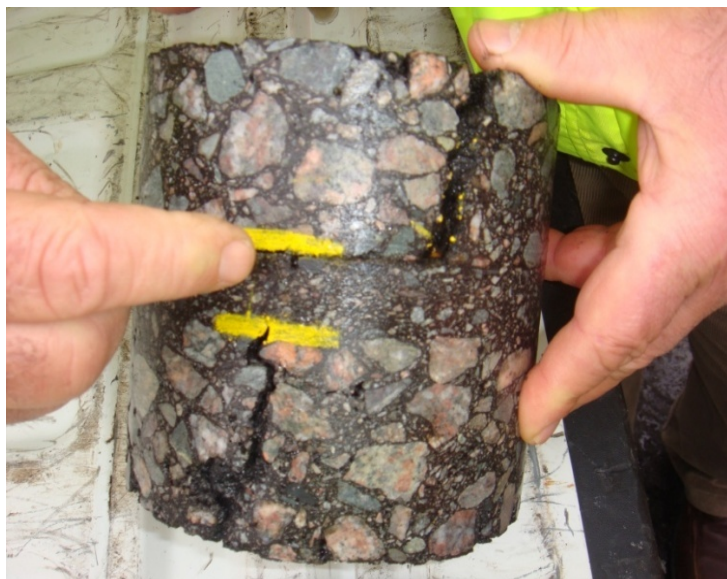
FIGURE 4 Cracking above and below a highly fatigue-resistant mixture.
