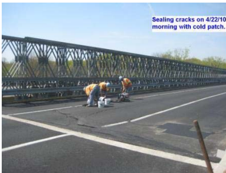
FIGURE 6 Patching of rapid deterioration on Route 80 ACROW bridge in New Jersey.
