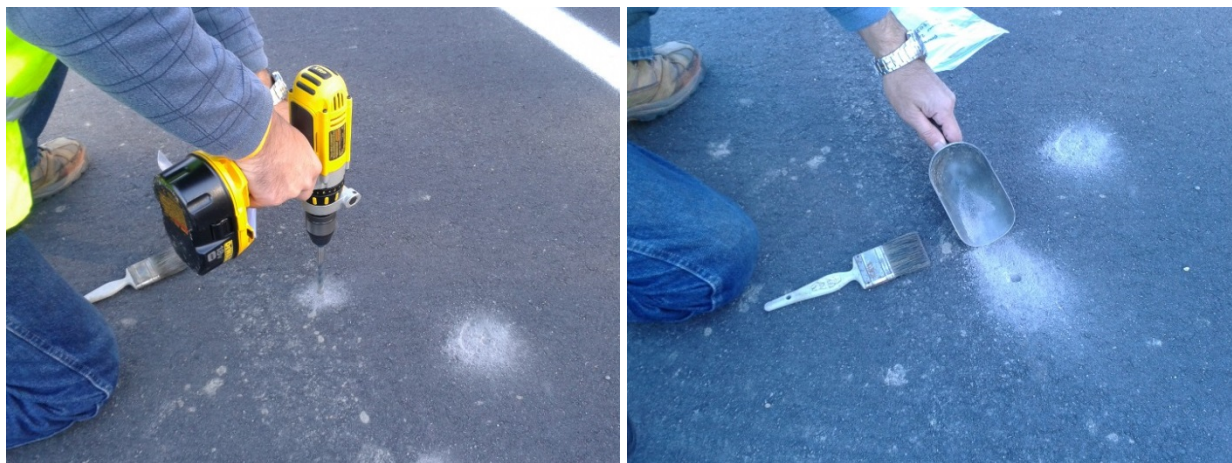
Figure B.6. Recovering an HMA sample from a pavement surface (left) and placing a pavement surface sample in a bag (right).
