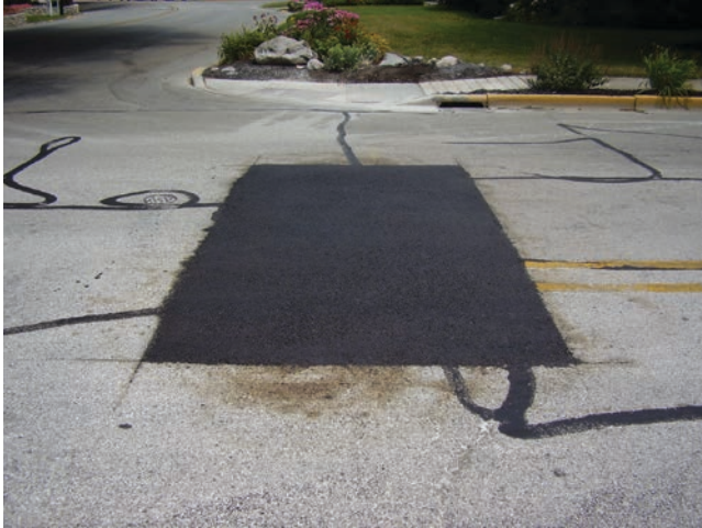
FIGURE 8 A semi-permanent patch on asphalt pavement (Source: R. McDaniel).
