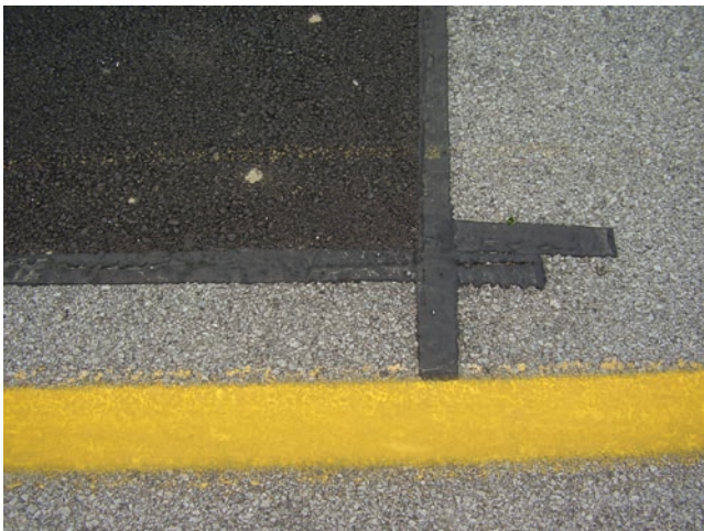
FIGURE 9 Excellent edge seal on semi-permanent asphalt patch (Source: R. McDaniel).
