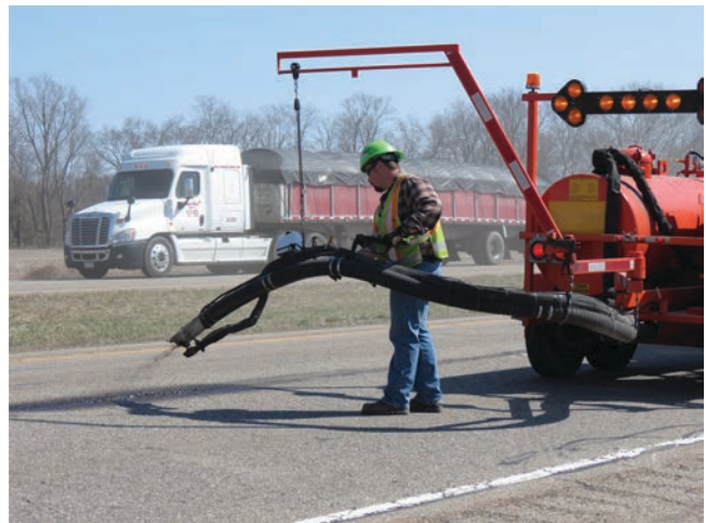
FIGURE 11 Patching with trailer-mounted spray injection patcher (Source: Ohio DOT).
