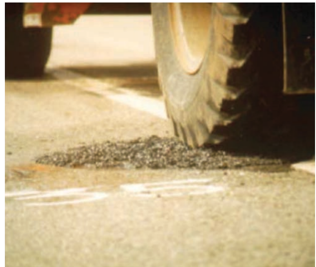
FIGURE 7 Rolling a patch with truck tires (Source: CLRP).
