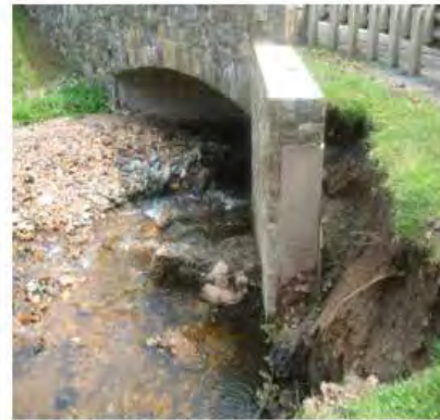
Rt 202 over Branch of Mine Brook, MP 35.42, Structure # 1809153, Bernardsville Boro. Somerset Co, washout & undermining
