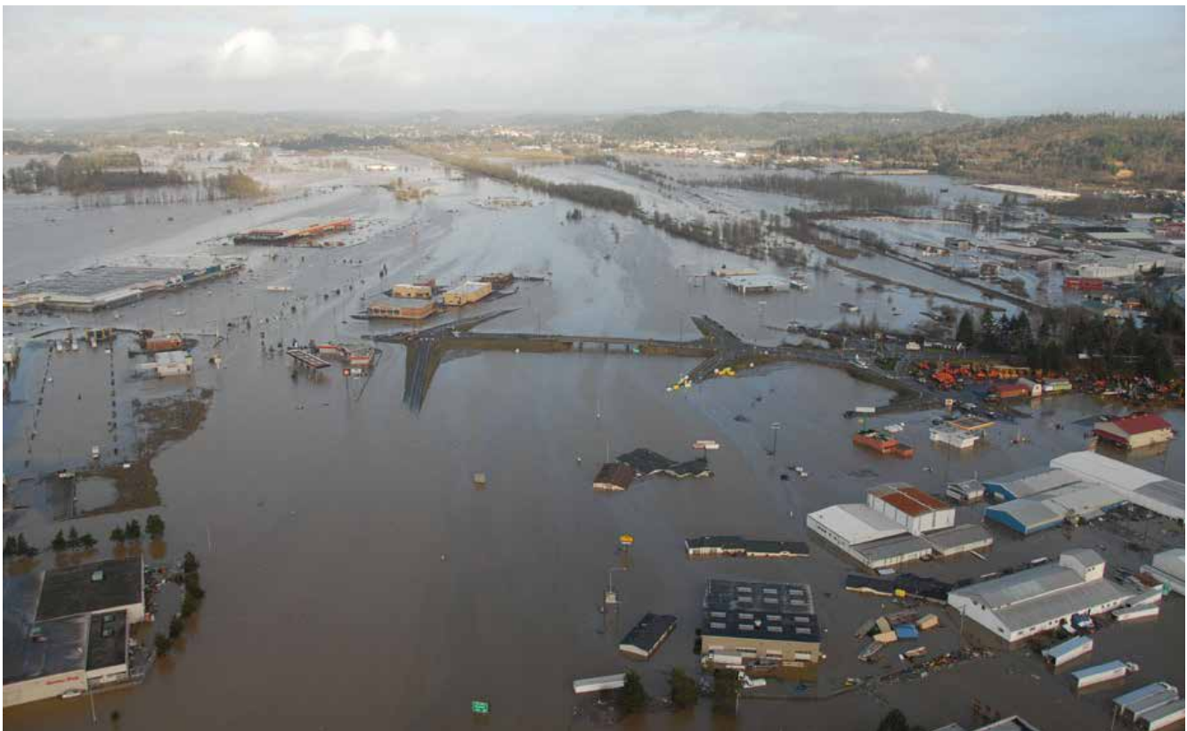
FIGURE 11 Aerial view of inundated Interstate 5, showing the freeway overpass in center of photo, Chehalis, Washington, December 4, 2007 (Flickr Commons, WSDOT).
