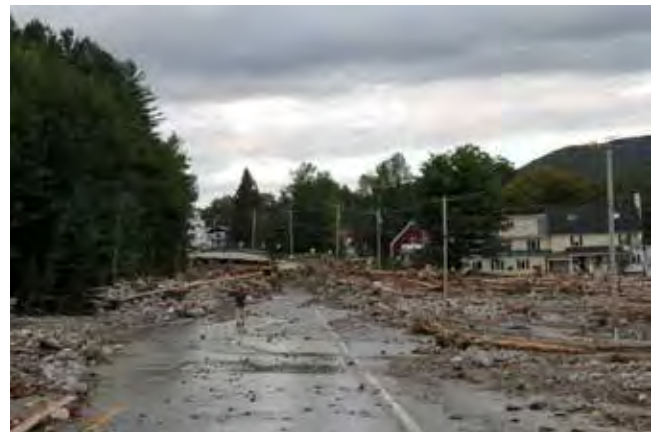
FIGURE 13 Tropical Storm Irene roadway damage and debris, Killington, Vermont, August 29, 2011 (Flickr Commons, Ashly Hauck).
