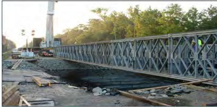
Rt 70,MP 20.40, EB & WVB, Str# 0310-154, Southampton Twp, Burlington Co.
