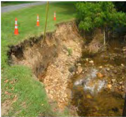
Rt 202 over Branch of Mine Brook, MP 35.42, Structure # 1809153, Bernardsville Boro. Somerset Co, washout & undermining
