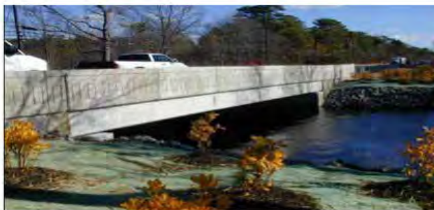
Rt 70,MP 20.40, EB & WVB, Str# 0310-154, Southampton Twp, Burlington County
