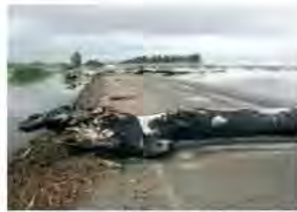
Debris on the roadway presented challenges after the water receded.
