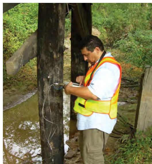
PHOTO: NORTH CAROLINA DOT
