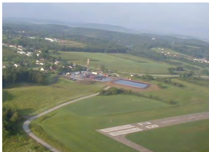
Figure 3.26. Drill pad and frack pond at Jimmy Stewart Airport, PA.
