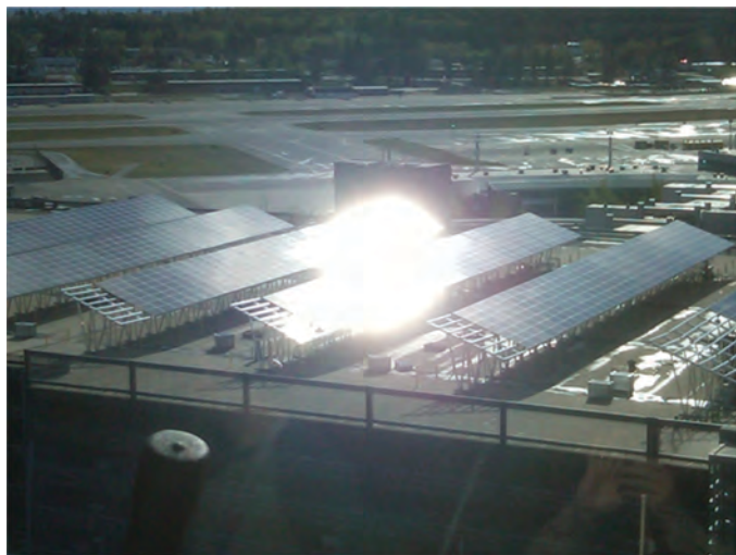
Figure 3.7. Glare viewed from MHT air traffic control tower.
