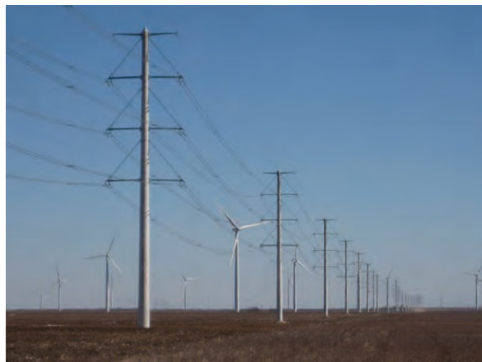
Figure 3.38. Recently constructed transmission lines as part of the CREZ project.
