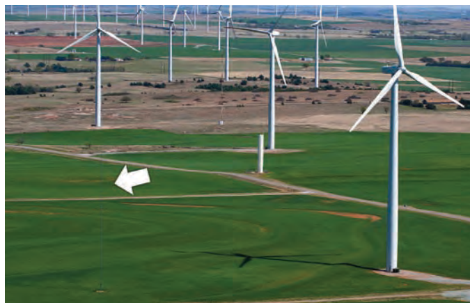
Figure 3.20. 198-foot MET within a wind farm array.
