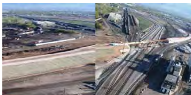
FIGURE 21 Ogden Yard ATC (Meyer et al. 2004).
