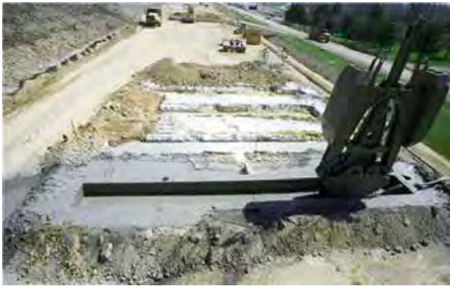
FIGURE 18 Jet grouting in progress (Trevicos 2010).
