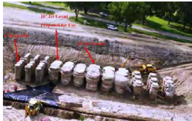
FIGURE 19 Jet-grouted samples prior to destructive testing (Note the size of the samples compared with the size of the equipment in the picture) (Hoffman et al. 2009).
