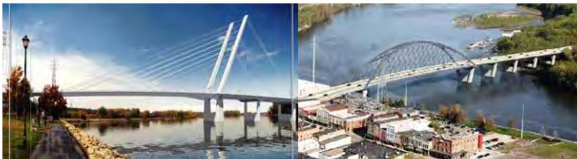
FIGURE 28 Unsuccessful proposal Hastings Bridge designs (Ravn 2012). (Note: Left is ATC design and right is the baseline design.)
