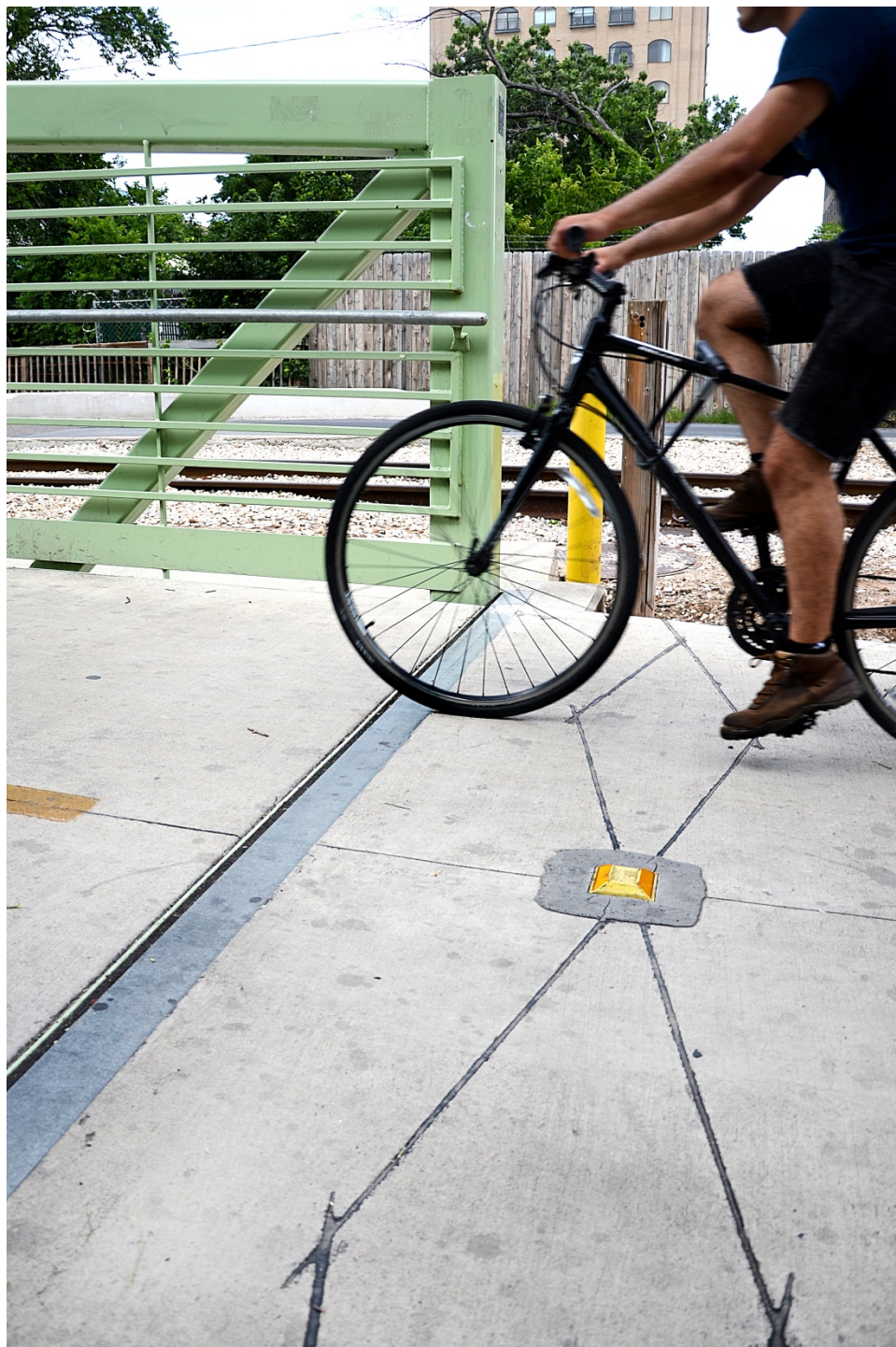
FIGURE 2 Inductance loops and infrared sensors detect bicyclists and pedestrians constantly on the Lance Armstrong Bikeway in Austin, Texas. (Photo: Jim Lyle, TTI.)
