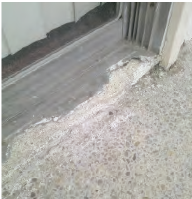
Figure 3-3. Damaged aluminum frame.
