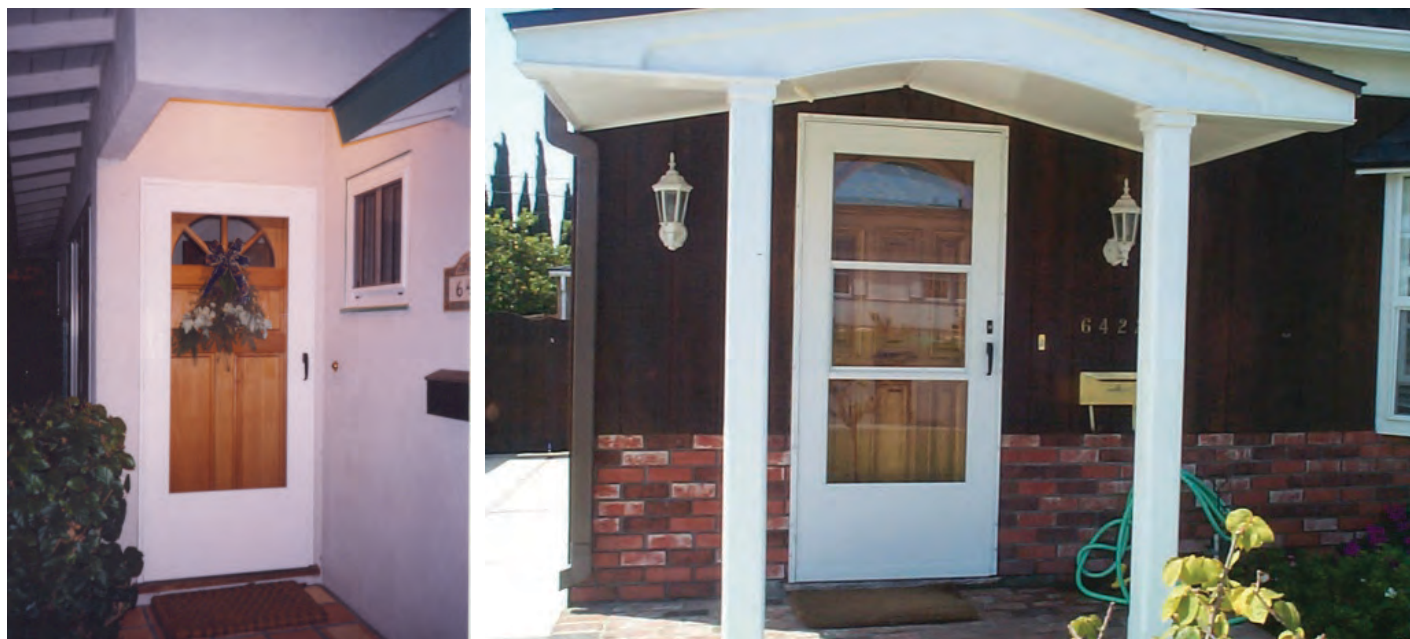
Figure 4-6. Full glass and self-storing storm doors.
