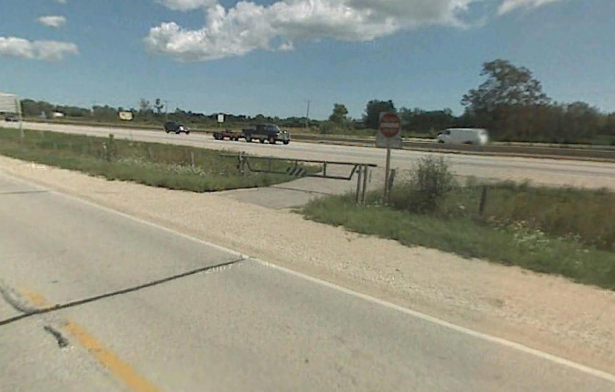
Figure 3.17. Emergency access between interchanges.
