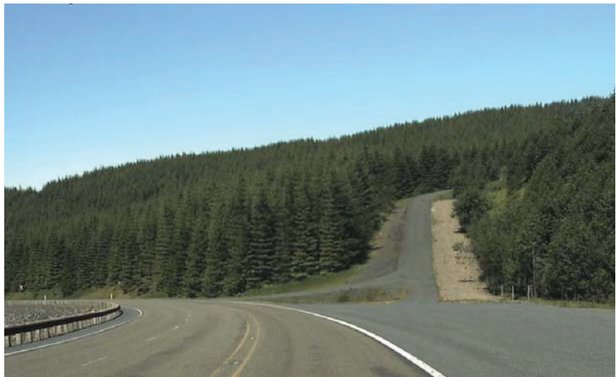
Figure 3.22. Runaway truck ramp. Source: Washington State Department of Transportation (2009).
