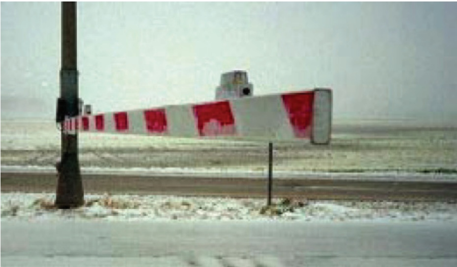
Figure 3.19. An automated gate used to close access in response to severe weather conditions.
