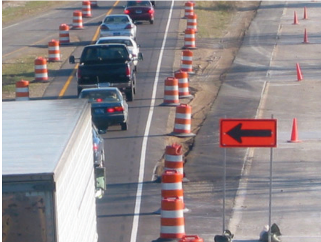
Figure 4.2. Traffic diverted across median. Source: Federal Highway Administration website.
