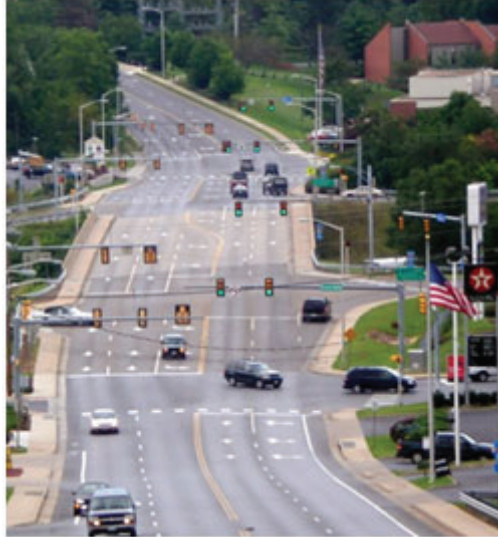
Figure 4.12. A series of traffic signals controlled by a signal timing system. Source: FHWA (2011).
