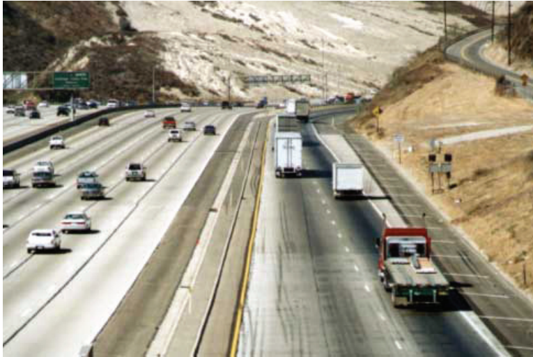
Figure 4.7. Interchange bypass lanes in Los Angeles, California. Source: Neudorff et al. (2003).
