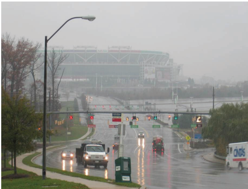
Figure 4.8. Reversible lane used for clearing stadium traffic in Baltimore, Maryland.
