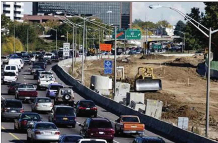
Figure 3.23. Construction project causing freeway congestion. Source: Knauer et al. (2006).
