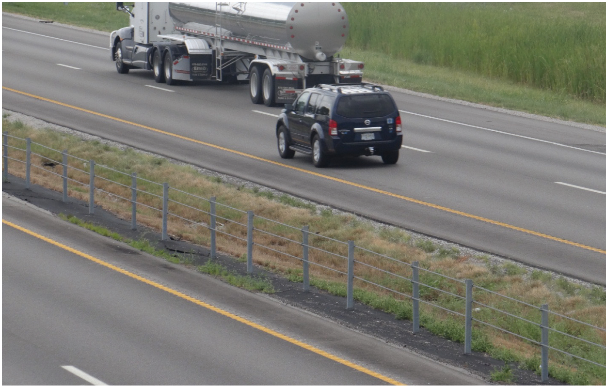
Figure 3.4. Standard three-strand movable cable median barrier.
