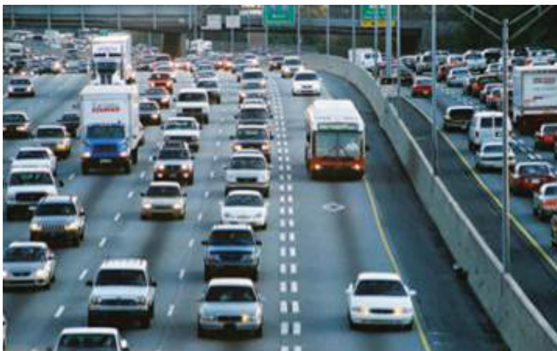
Figure 4.6. HOV lane in Atlanta, Georgia. Source: Transportation Conformity Brochure (FHWA 2010).
