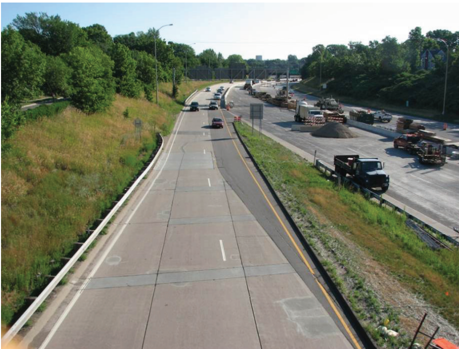
Figure 3.18. A two-lane off-ramp in Minnesota.
