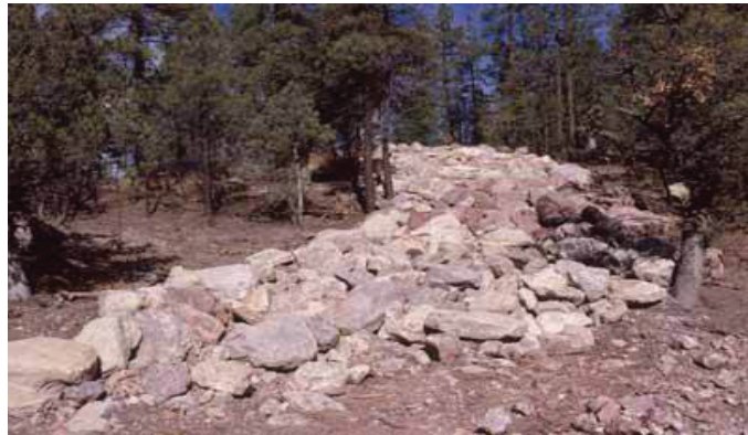
Figure 3.25. Boulders in the right-of-way (alternative to wildlife fencing). Source: Huijser et al. (2008).
