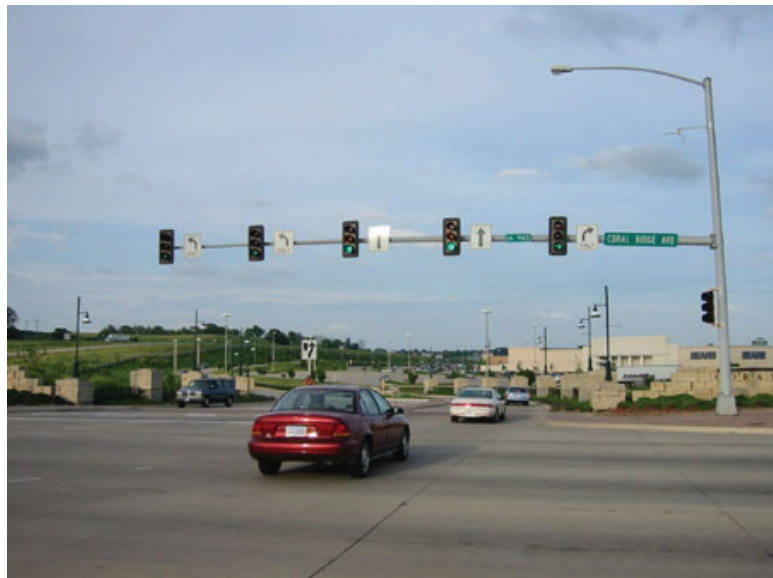
Figure 4.11. Lane-aligned signal heads. Source: Rodegerdts et al. (2004).
