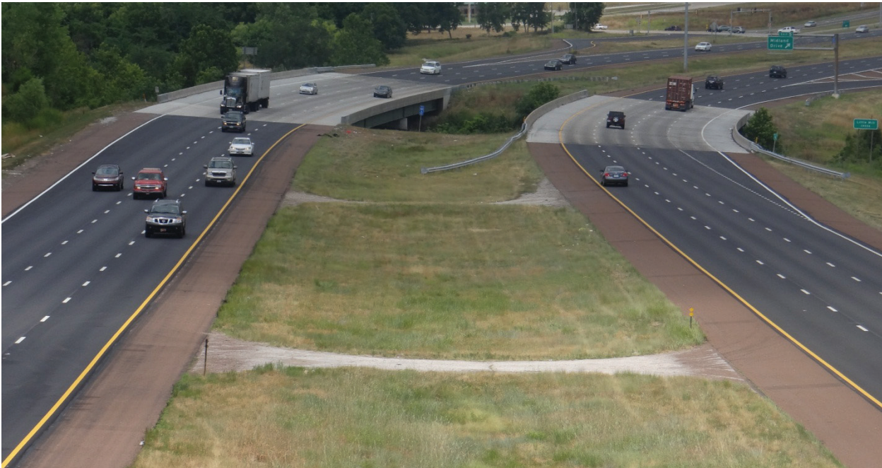
Figure 3.1. Emergency crossover on I-435 in Kansas.
