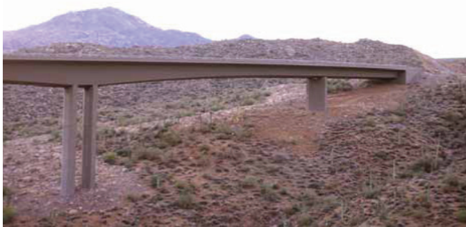
Figure 3.26. Long tunnels and long bridges physically separate animals from vehicular traffic.
