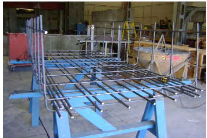
Figure C.9. Bottom cage reinforcement.
