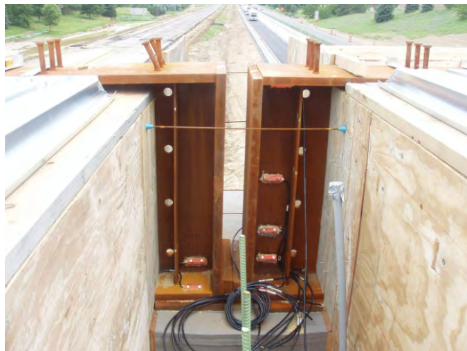
Figure B.8. Continuity without top flange splice.
