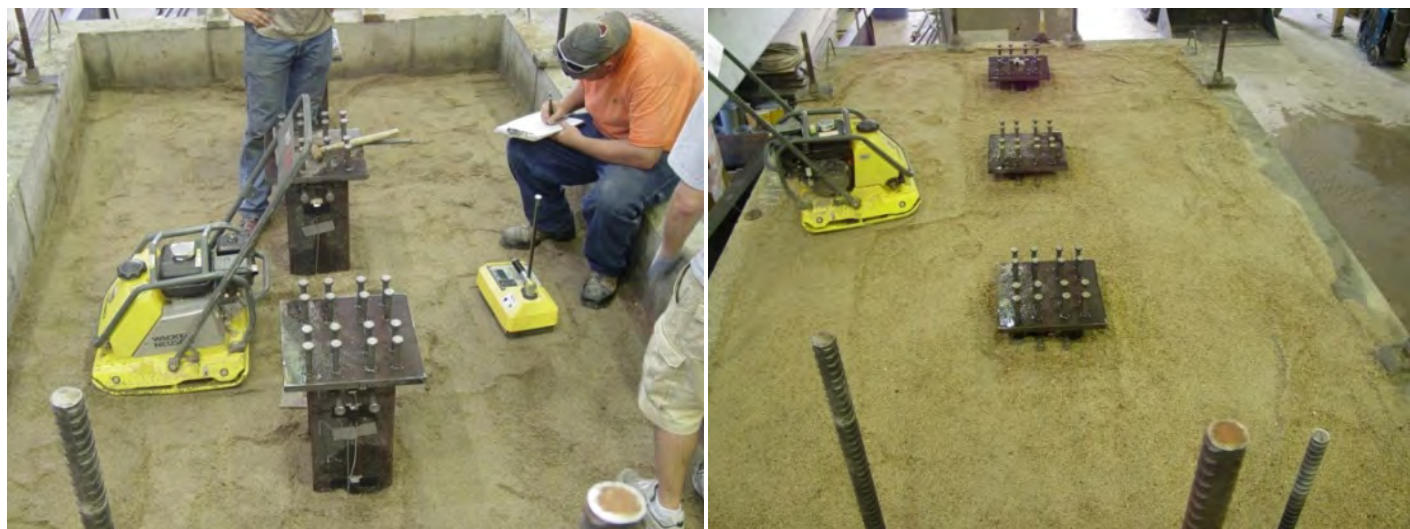
Figure 3.56. The relative density of the compacted soil is measured using a nuclear density device.
