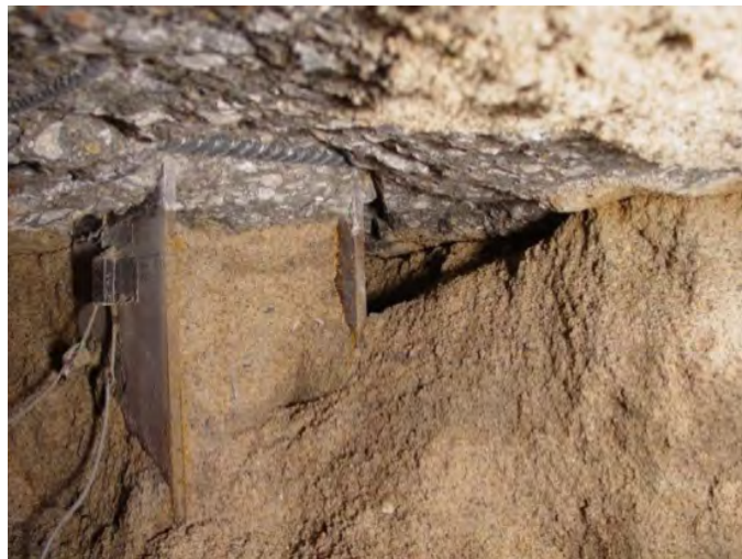
Figure 3.59. Compaction of CDF around a small pile.
