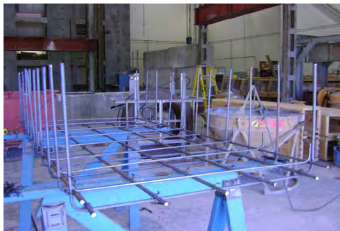
Figure C.10. Top cage reinforcement.
