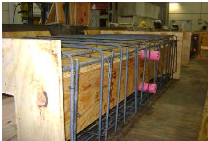
Figure C.11. Box girder without side forms.
