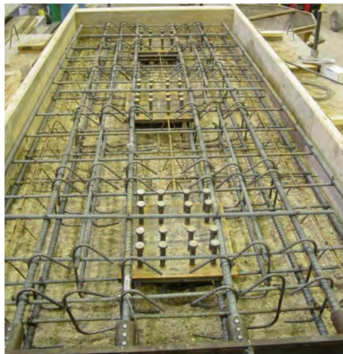
Figure 3.57. Reinforcement of the top slab.
