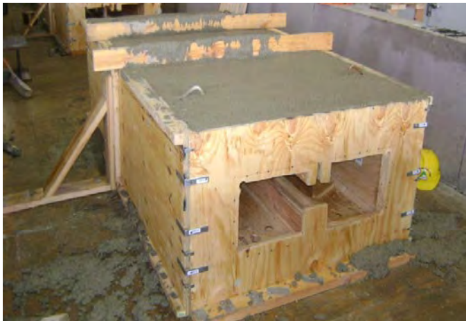
Figure C.12. Box girder immediately after casting.
