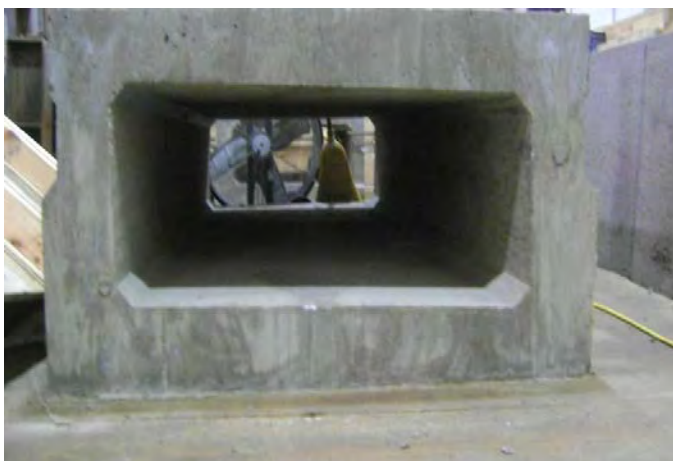
Figure C.13. Box girder without interior and exterior forms.
