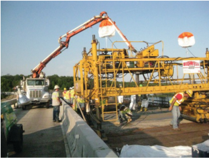
Figure F.5. Pump truck.
