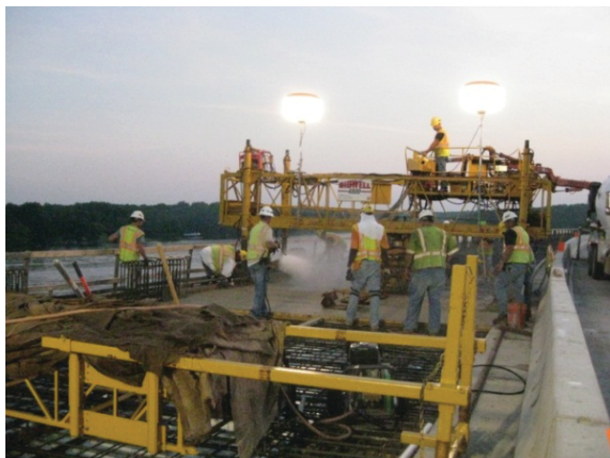
Figure F.7. Water being sprayed on surface.
