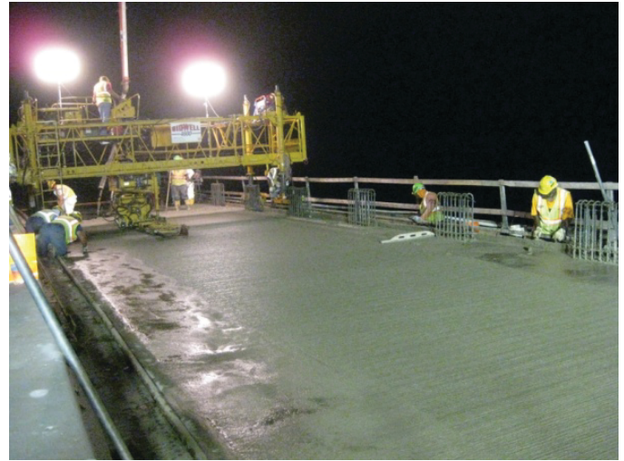
Figure F.8. Hand finishing.
