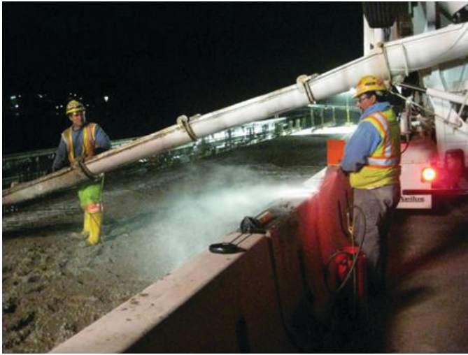
Figure F.2. Water sprayed on concrete using the truck hose.
