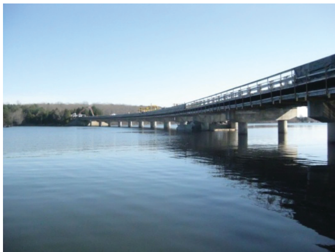
Figure F.1. Route 208 bridge over Lake Anna.
