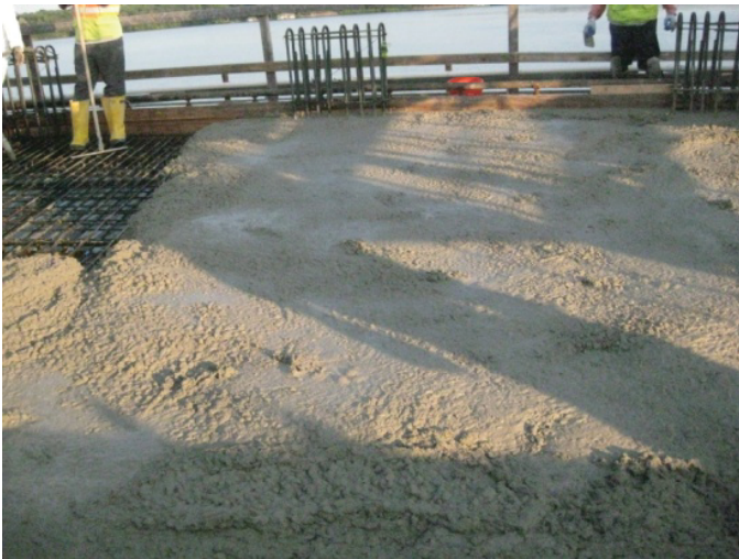
Figure F.6. Vibration brought fine material to the surface.
