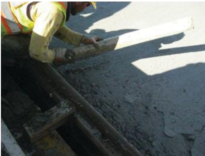
Figure F.3. Extra paste worked into the surface.
