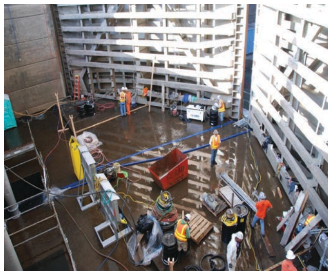
Figure 5.2. The Dalles Lock repair, 2009.
