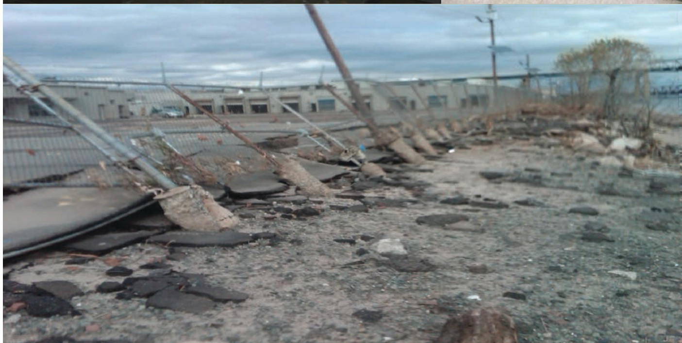
Figure 4.7. Flooding at port terminal buildings and damage to security fencing.
