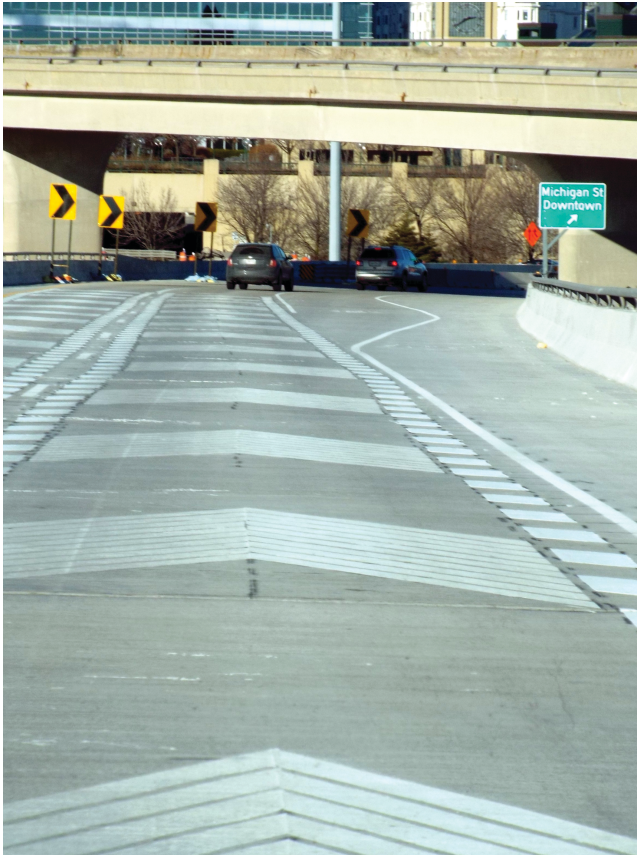
FIGURE 29 Converging chevron pattern at a 2014 Wisconsin work zone.
