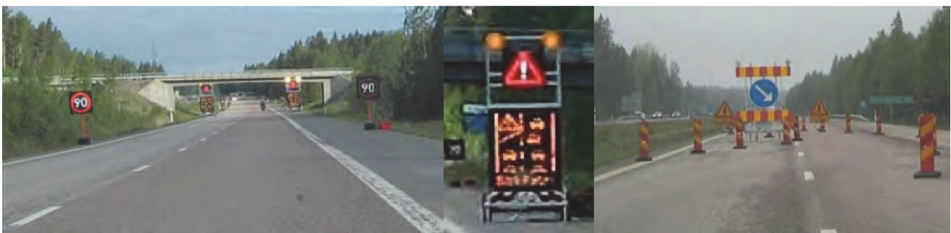
FIGURE 54 Swedish upstream chicane marking enhanced with LED/VMS signage (Nygårdhs 2007).
