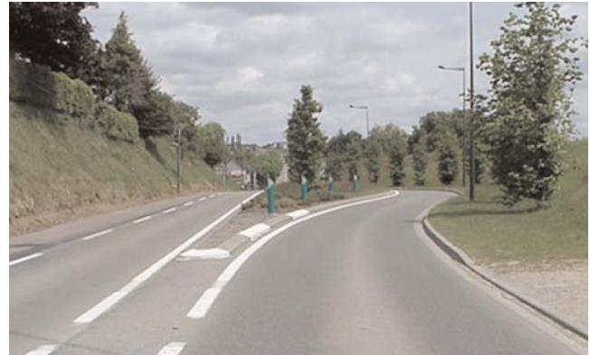
FIGURE 17 Permanent chicane intended to reduce speeds on highway D29 on a downgrade entrance to the village of Ernée, Mayenne, France (CERTU 2006, 2007).
