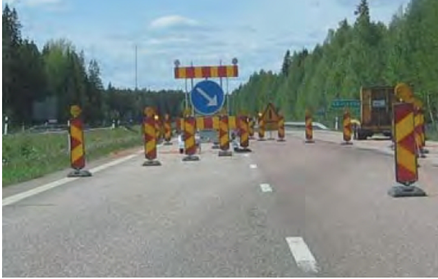
FIGURE 21 Approach to chicane at a rural freeway work zone in Sweden (Nygårdhs 2007).
