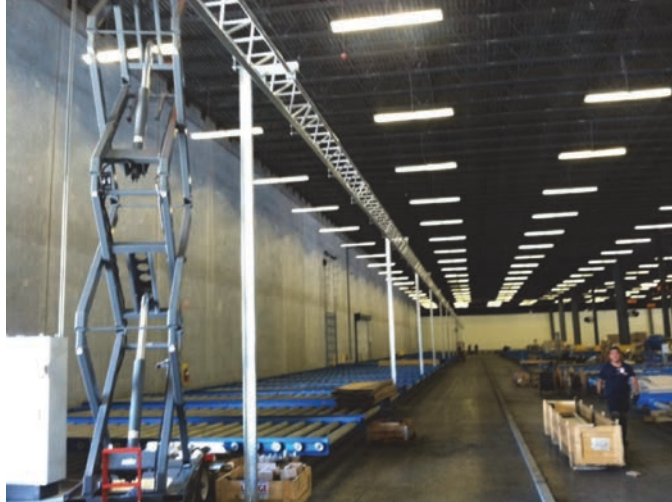
Figure 4-18. ETV system being installed at Centurion air cargo facility.
