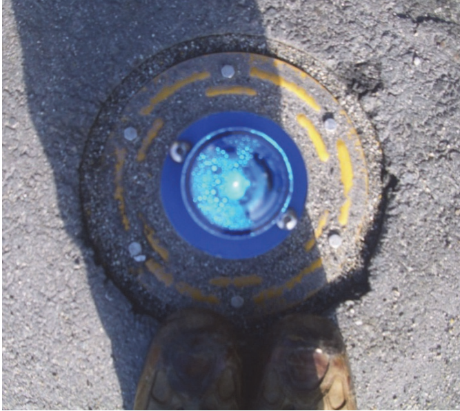
Figure 25. Moisture build-up inside fixture.
