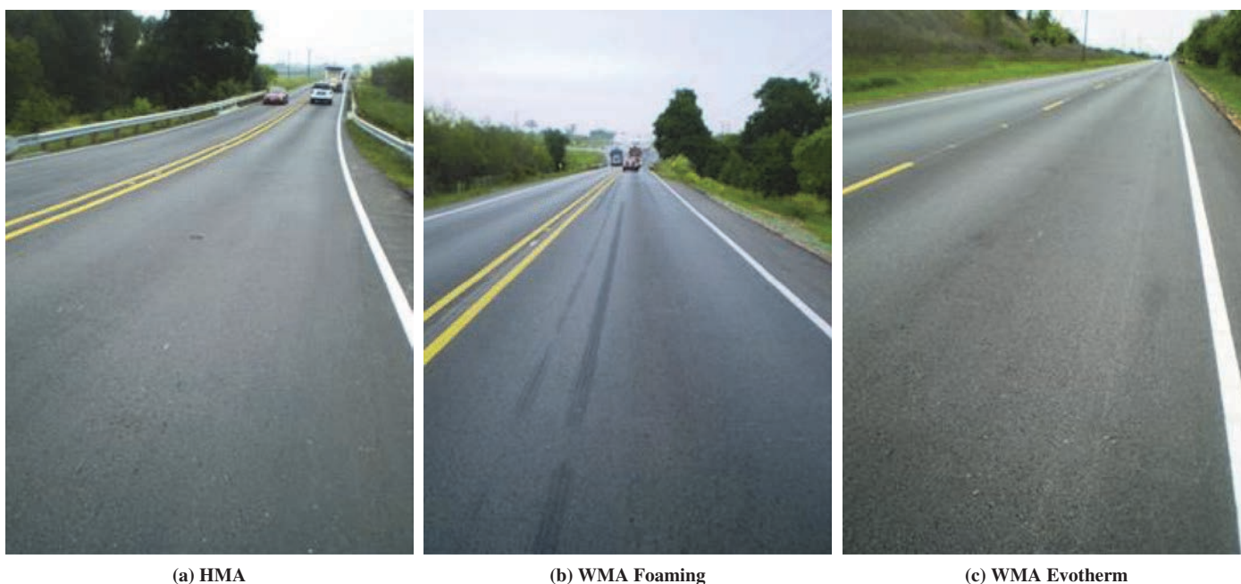
Figure A-11. Performance of the Texas field sections after 2 to 3 months in service.
