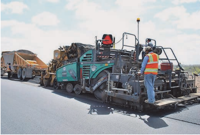
Figure A-64. Paving with windrow operation at the Midland–Odessa field site.
