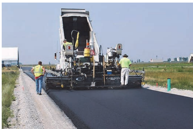
Figure A-41. Paving of surface layer at Central Iowa Expo Center.
