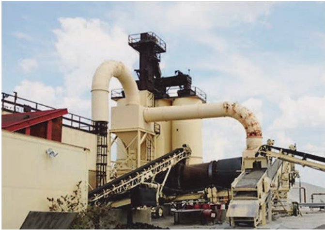
Figure A-52. Rieth-Riley's counter-flow drum plant in Indianapolis, Indiana.
