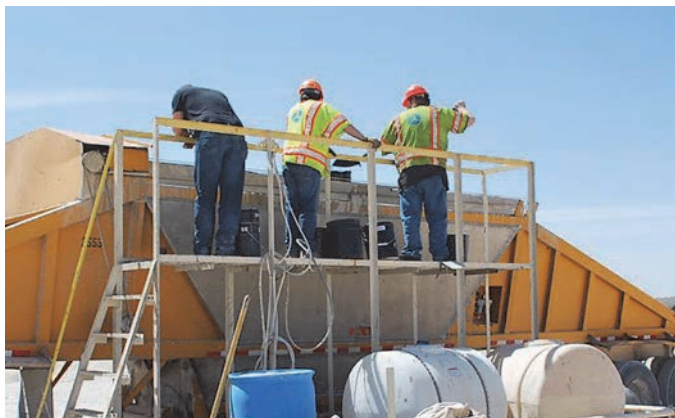
Figure A-66. Loose mix sampling from truck in Midland–Odessa drum plant.
