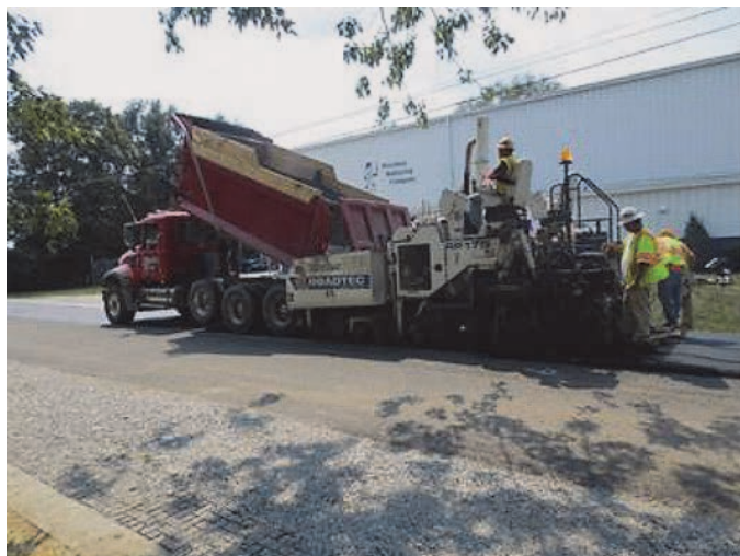
Figure A-56. RoadTec paver used in Indianapolis, Indiana.
