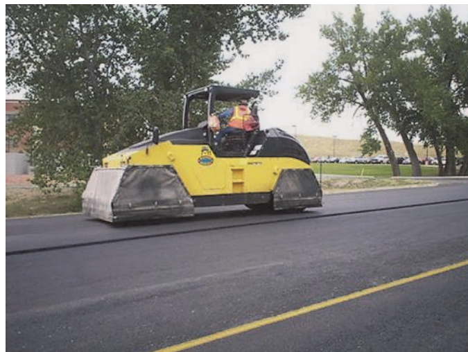
Figure A-28. Compaction using pneumatic roller.
