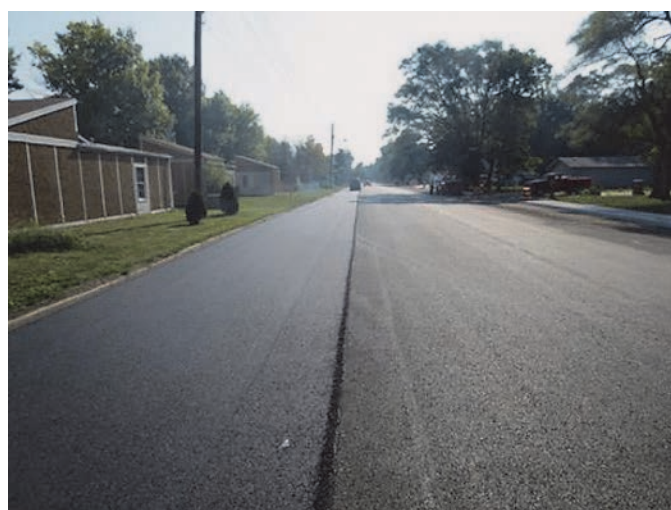
Figure A-58. Example of compacted HMA (batch plant).
