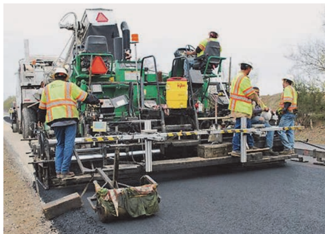
Figure A-7. Paver equipped with PAVE-IR bar.
