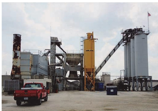
Figure A-51. Rieth-Riley's modified batch plant in Indianapolis, Indiana.
