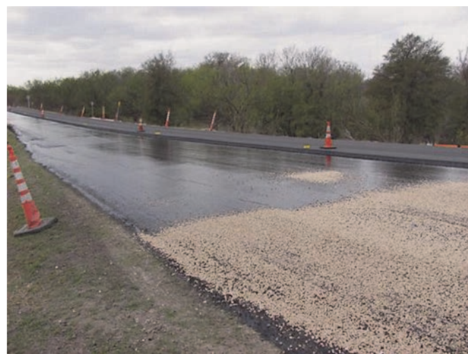
Figure A-5. Application of underseal before overlay laydown.
