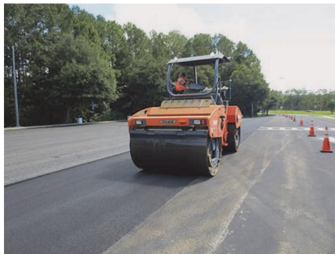
Figure A-48. Breakdown roller compacting granite HMA.
