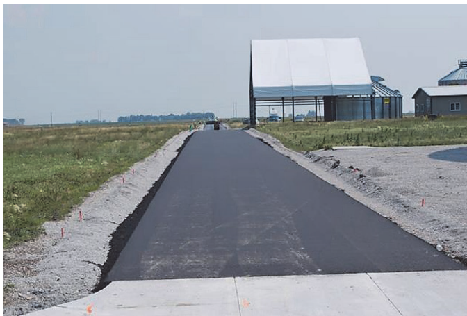
Figure A-36. Typical test section at Central Iowa Expo Center.
