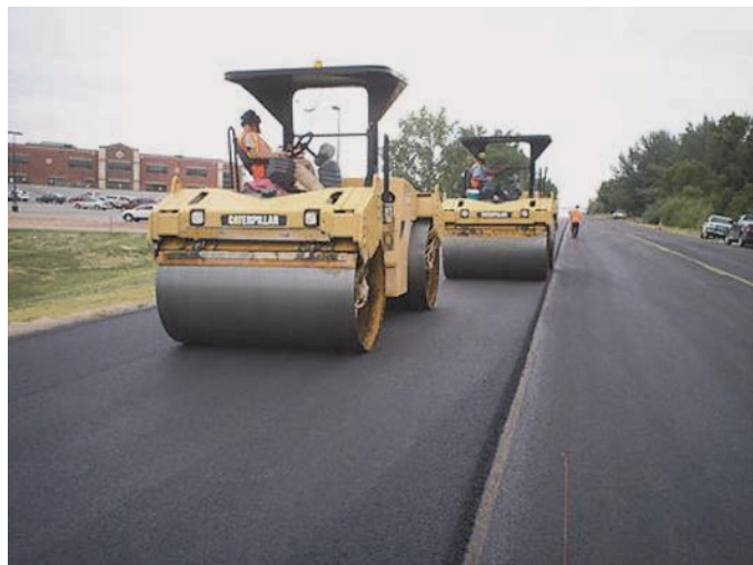
Figure A-27. Breakdown with vibratory rollers.
