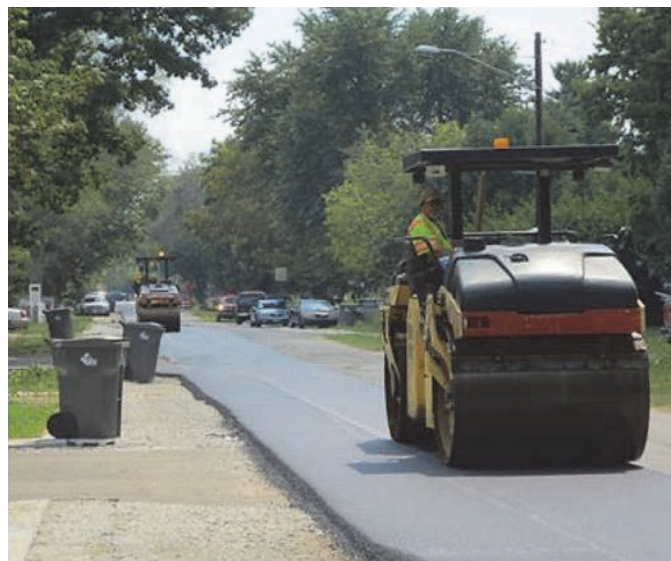
Figure A-57. Breakdown and finishing rollers compacting the HMA drum mix.
