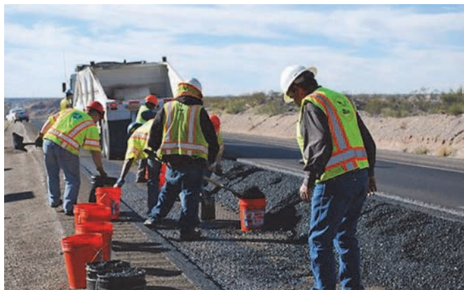
Figure A-19. Loose mix sampling at the New Mexico field site.
