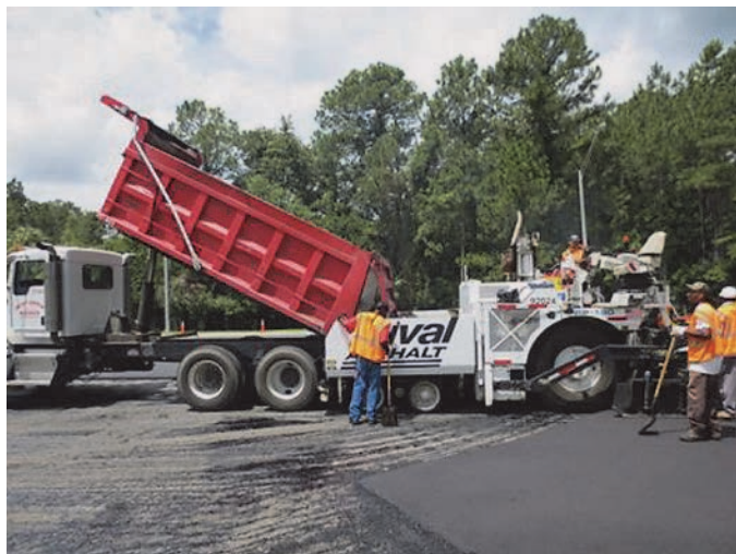
Figure A-47. RoadTec paver used in Jacksonville, Florida.
