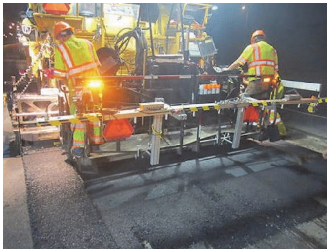
Figure A-23. Paver equipped with PAVE-IR bar.
