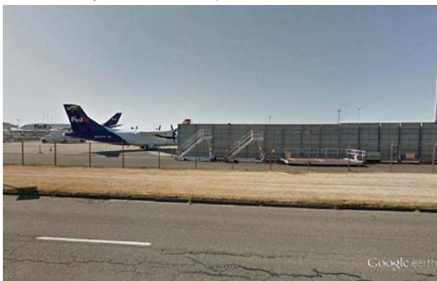
Figure 9-21 Air Cargo Ramp Jet Blast Fence at SEATAC International Airport. (SOURCE: Google Earth Pro, CDM Smith.)
