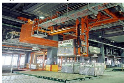
Figure 9-27 Examples of Automated Terminals and Gateways. (SOURCE: Lynxs Group.)
