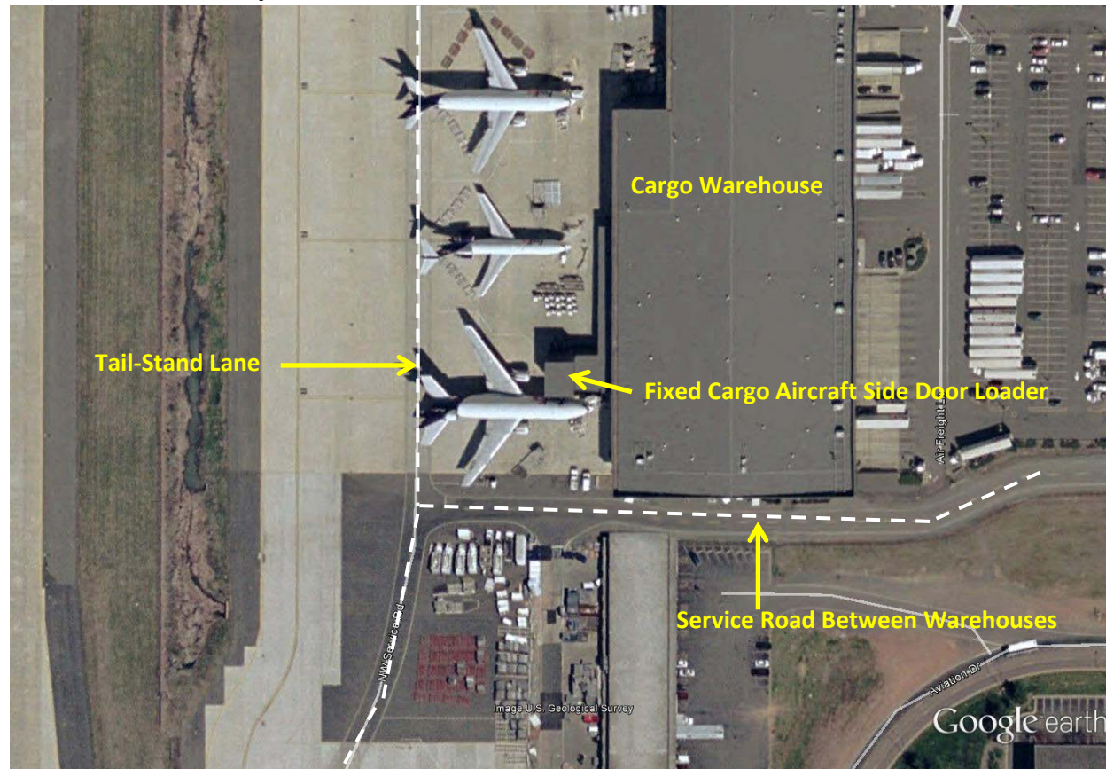
Figure 9-19 Roads between Cargo Warehouses and Apron Configuration. (SOURCE: Google Earth Pro, CDM Smith Analysis.)
