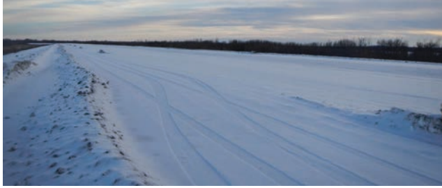
FIGURE 23 Typical snow removal equipment building used at Alaskan rural airports. Photo credit: J. Worrall, Alaska DOT&PF.
