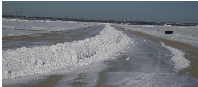
FIGURE 13 Example of snow having been windrowed to allow for a snowblower to remove it. Photo credit: C. Lawson, Romeoville, Illinois.
