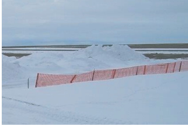
FIGURE 17 Example of a snow fence installed at an airport. Photo credit: J. Moline, Lewistown, Montana.
