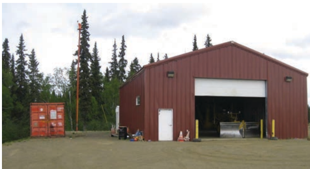
FIGURE 24 Example of frozen gravel berms surrounding light fixtures at Alaskan rural airports. Photo credit: J. Worrall, Alaska DOT&PF.
