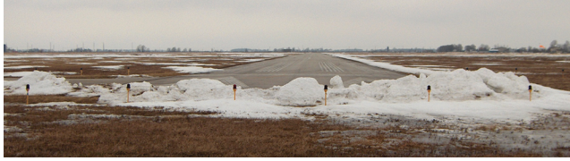
FIGURE 11 Example of hazardous snowbanks at a runway approach. Photo credit: S. Quilty, SMQ Airport Services.
