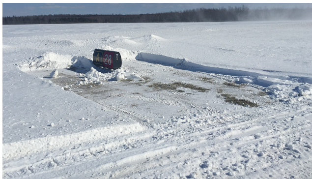
FIGURE 14 Example of using a snowblower to eliminate snow accumulations around lights and signs. Photo credit: G. Sussey, Watertown, New York.
