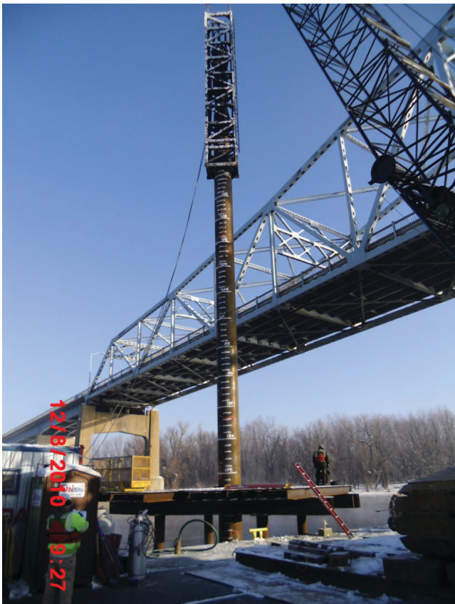
FIGURE 16 Driving Pier 6 test pile.
