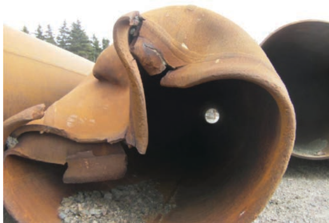
FIGURE 6 Buckling at the toe of steel LDOEP (courtesy: Bengt Fellenius).
